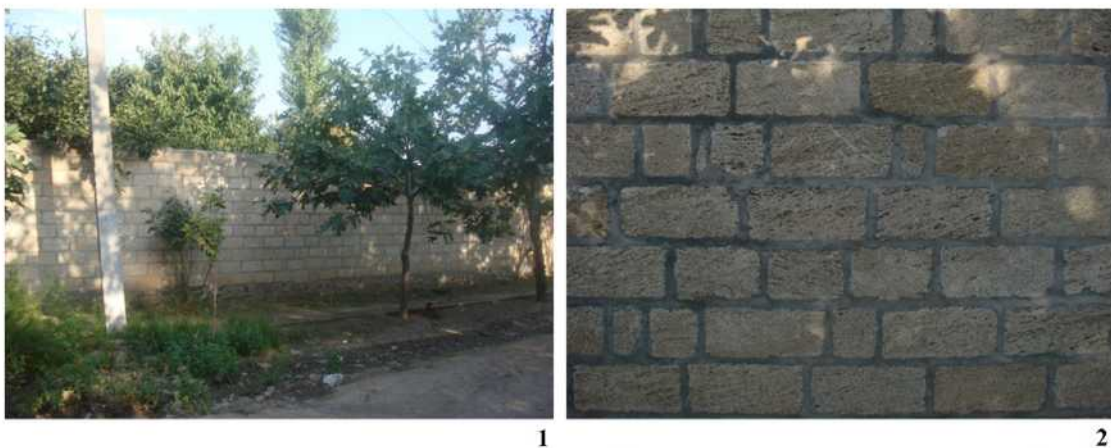
Fig. 6.5 Modern stone block wall in Qovlar Village, Tovuz, Azerbaijan. 1: General view; 2: Close-up view. Note the large variability in block length visible on the wall surface.
