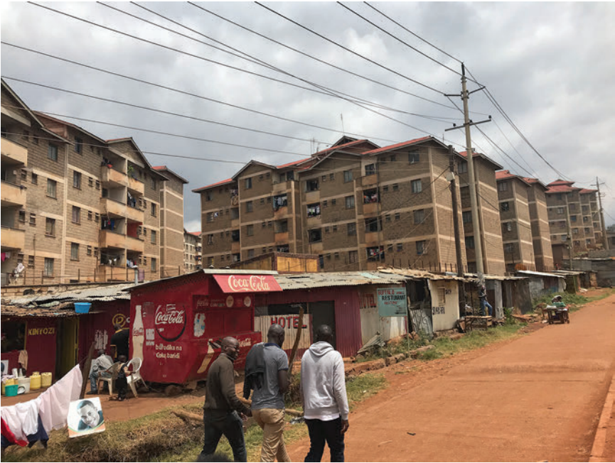
Fig. 4.5. Housing Conditions in Langata Decanting Site
