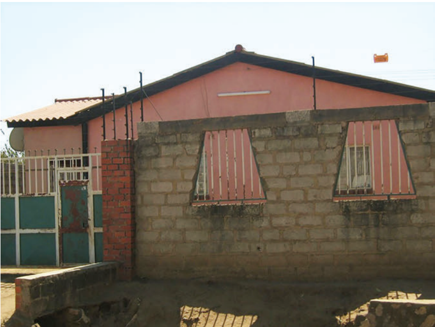
Fig. 7.3. Extended House in Matero
