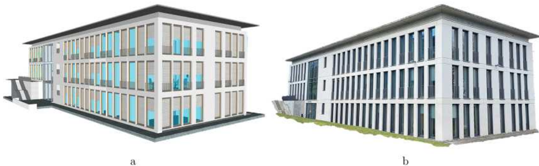
Figure 5.1: ITA-Building – Selected work site for verification of airborne sound insulation model (VBA Framework) (a) Virtual Building, (b) Real Building
