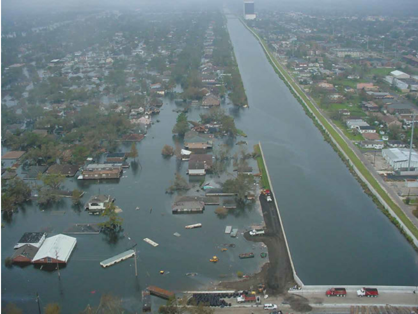
Figure 5.2. View of the 17 th Street Breach, Lakeview on the left. US Army photograph in the public domain. https://commons.wikimedia.org/wiki/File:New_Orleans_17th_Street_Canal_filling.JPG
