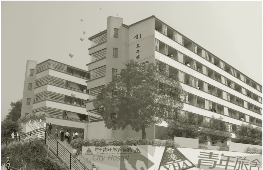
Figure 9.2 Artist's impression of the future Mei Ho House's front view (Commissioner for Heritage's Office 2010e) (with permission from Hong Kong Youth Hostels Association)
