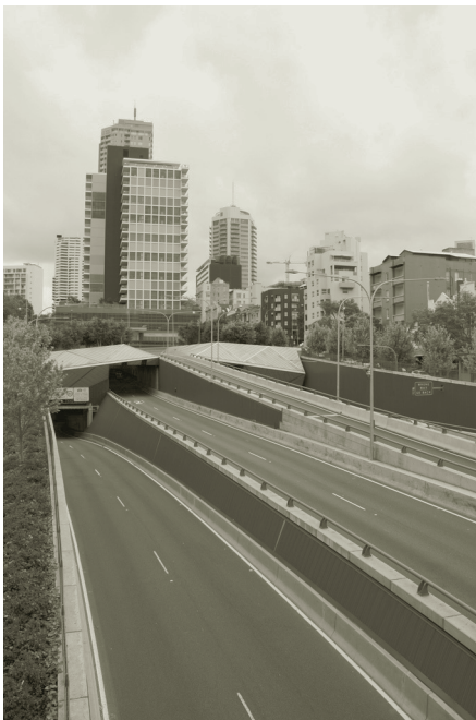
Figure 10.1 Photograph of the Cross City Tunnel (Judd 2008) (with permission from Trafford Judd)
