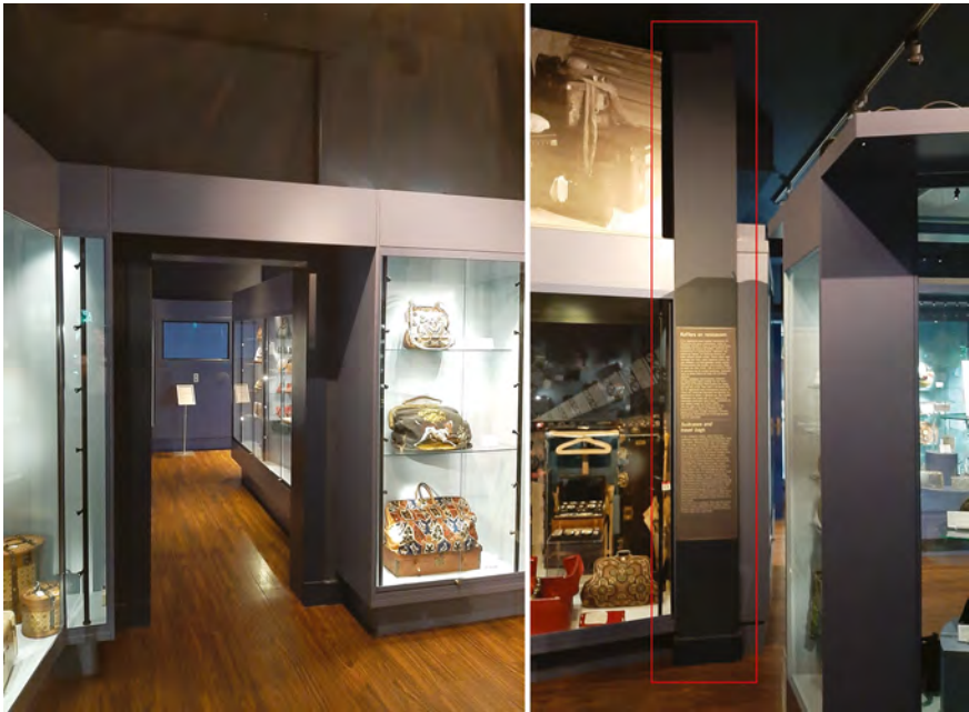
FIGURE 6.1 Pictures of the remaining walls which originally enclosed the boeken kamer , taken in 2019 by the author when the building hosted the Museum of Bags and Purses. Left: the wall and the original door opening which connected the library to the groene kamer . Right: Highlighted in red, the last standing part of the wall that divided the room from the grote kamer
