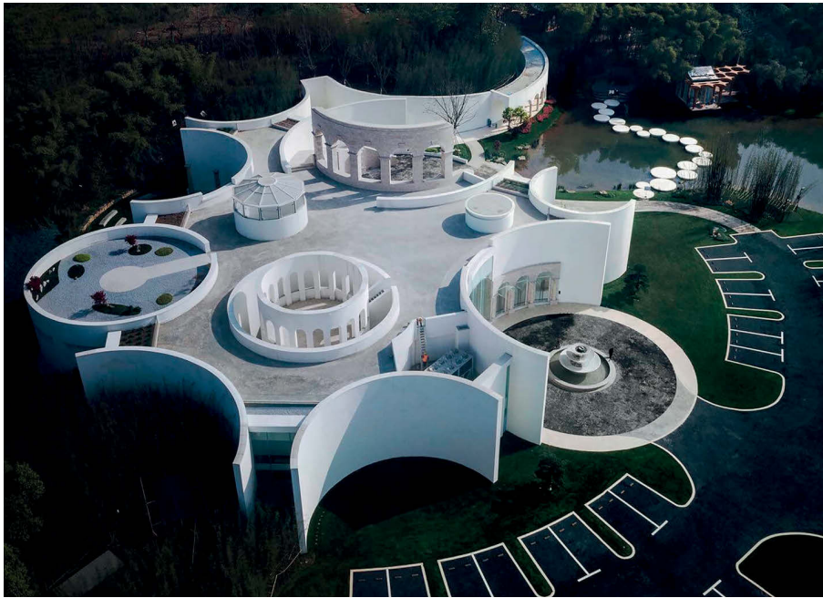
Circular walls, arcades, and skylights reminiscent of Classical aesthetics compose the Italian pavilion.
