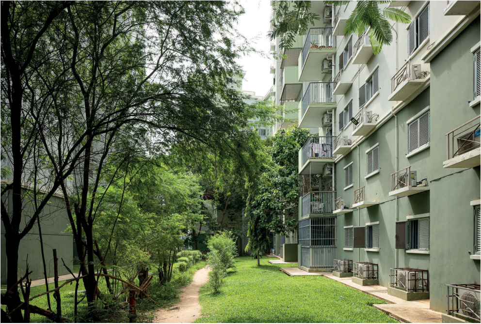
Relationship between the building's ground floor and the communal garden in Kilamba Kiaxi Housing Estate, Kilamba, Angola.
