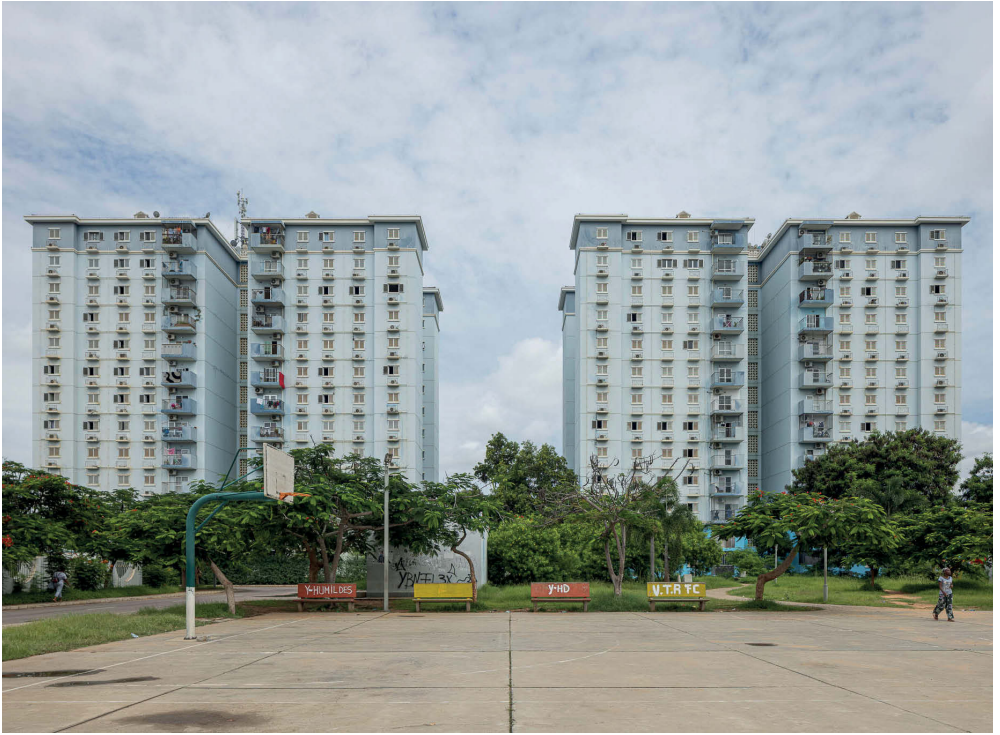
Communal space in front of new residential buildings within Kilamba Kiaxi Housing Estate, Kilamba, Angola.
