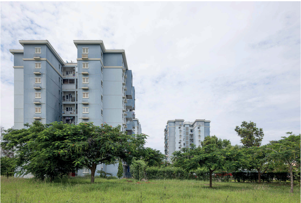
Relationship between the residential buildings and the surrounding natural landscape of Kilamba Kiaxi Housing Estate, Kilamba, Angola.
