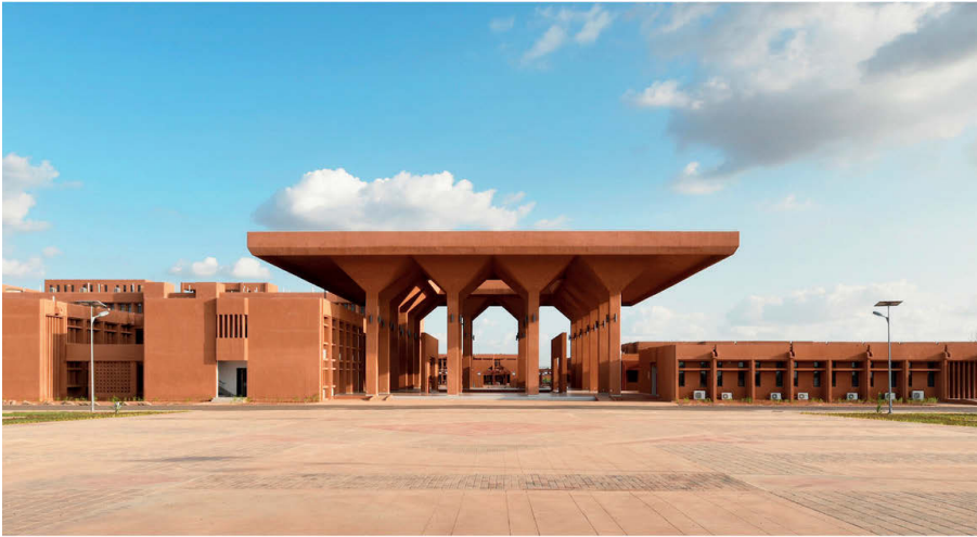
The main entrance is characterized by square-based columns connected to a perforated roof by trapezoidal elements.
