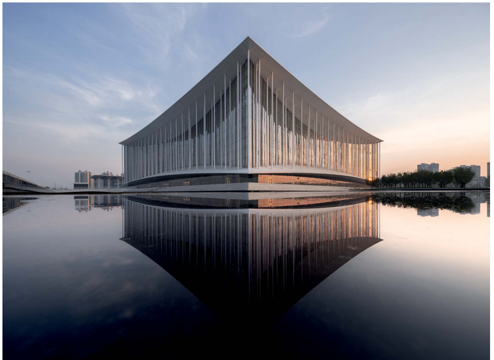
External structure made of two symmetrical horizontal vaults and several columns of the Xi'an Silk Road International Exhibition Center, Xi'an, China.
