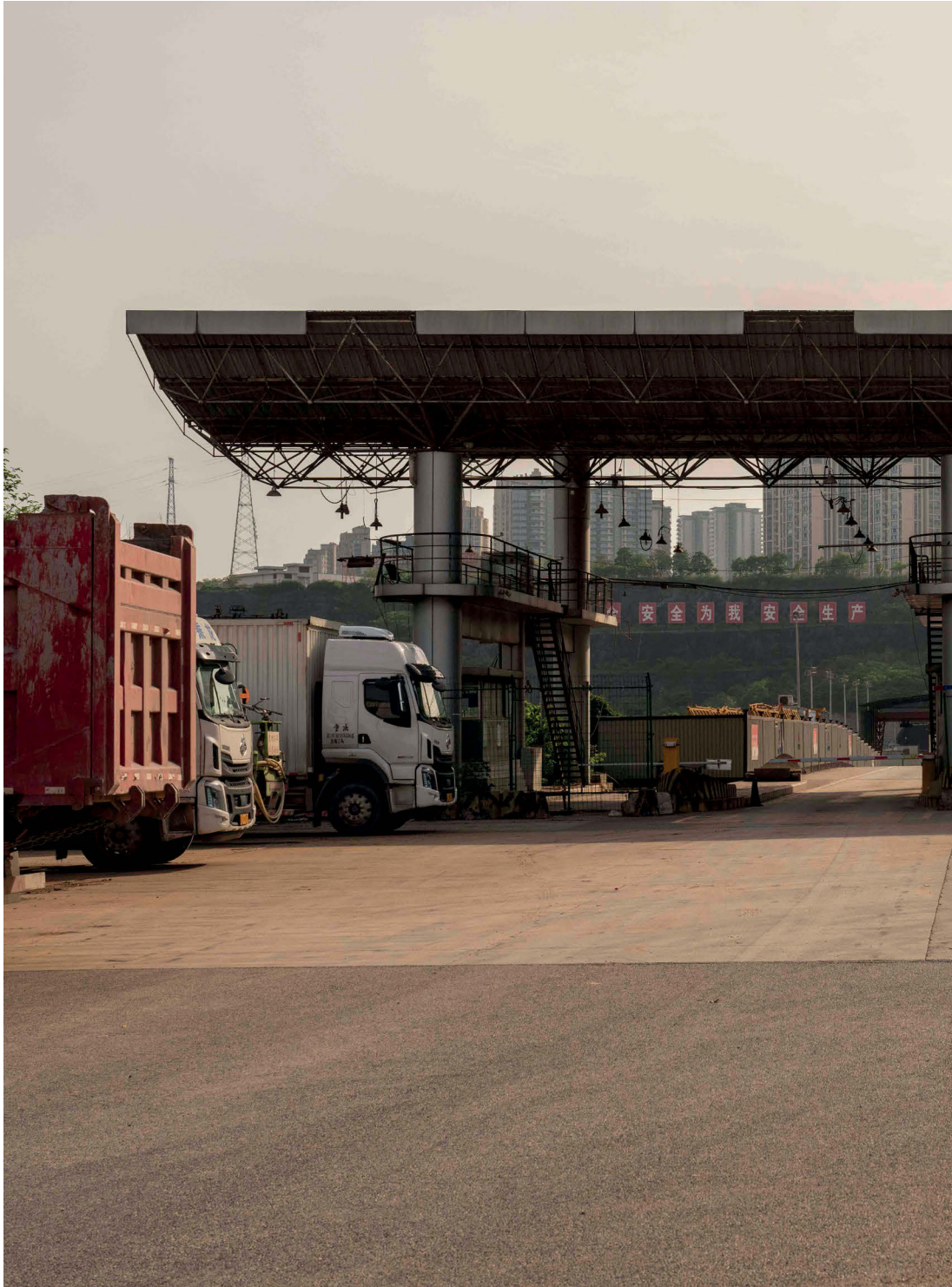
Main vehicular entrance to the Lianglu-Cuntan Free-Trade Port Area, Chongqing, China.
