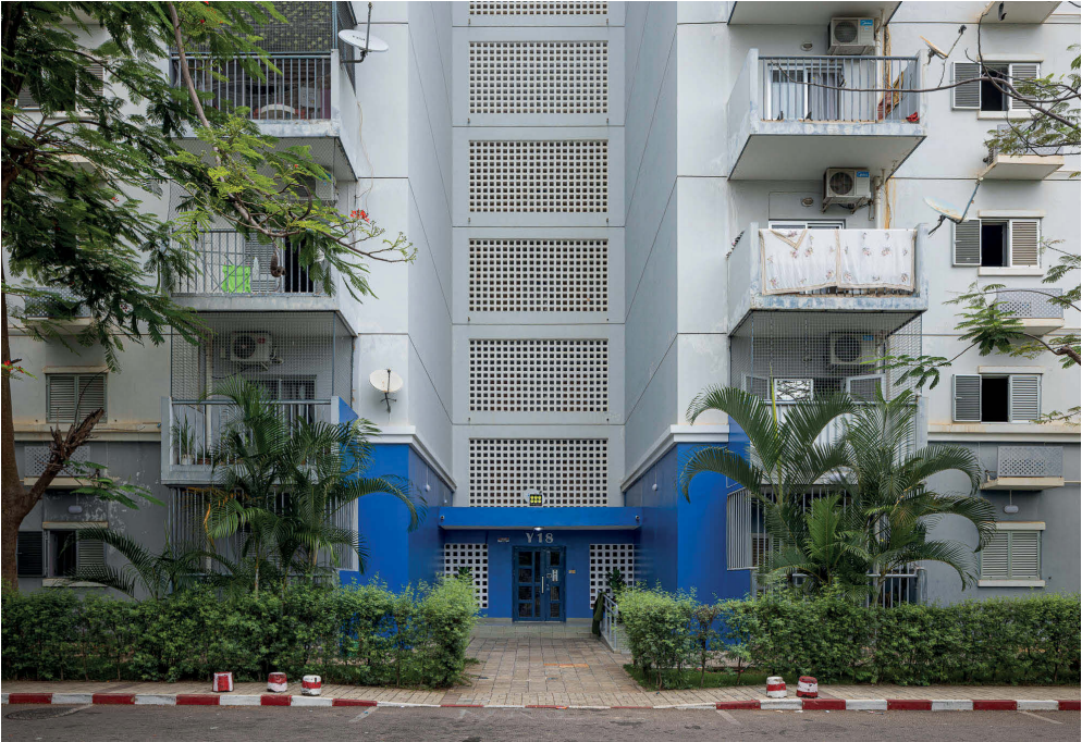
Lattice wall covering the distribution core of high-rise buildings in Kilamba Kiaxi Housing Estate, Kilamba, Angola.
