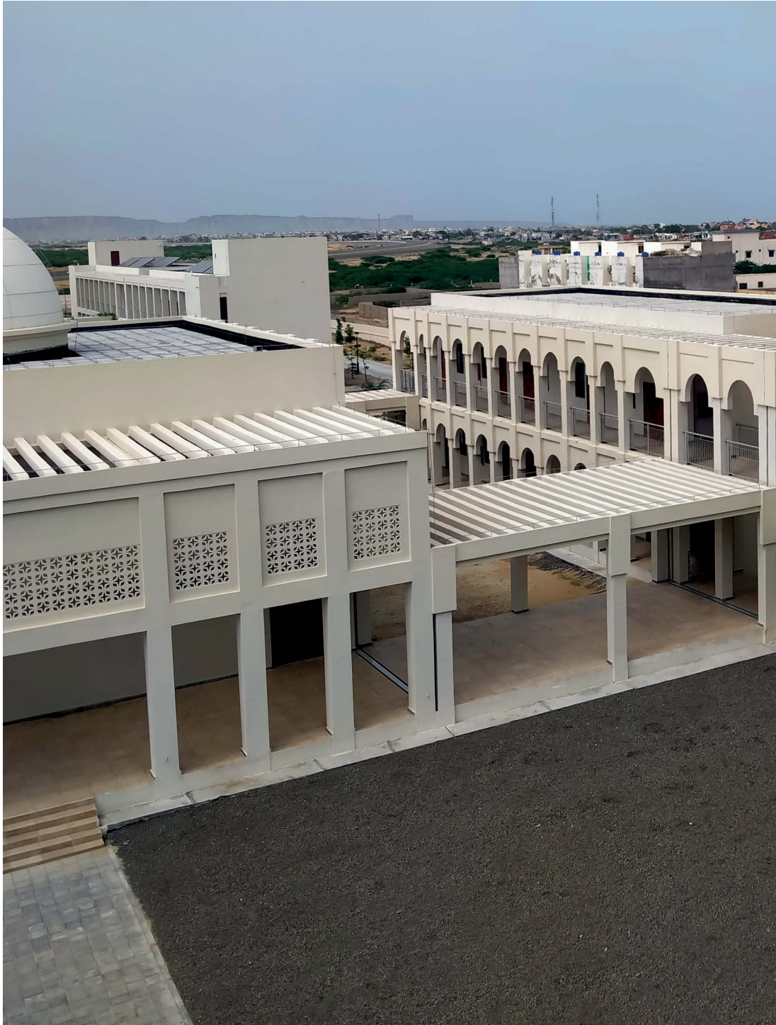
Main courtyard surrounded by arched porches in the Pakistan-China Technical and Vocational Institute, Gwadar, Pakistan.
