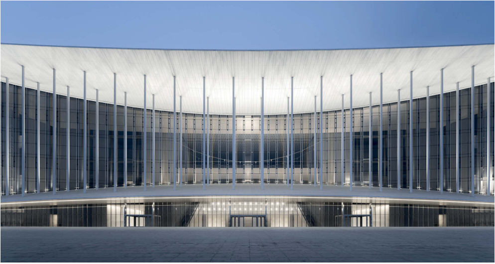
Mullion curtain wall of the Xi'an Silk Road International Exhibition Center, Xi'an, China.
