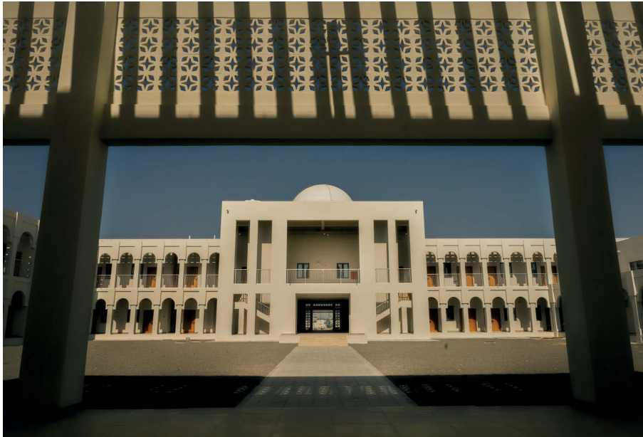
The main façade is characterized by a dome and a repetition of rounded arches inspired by the Gwadar vernacular mud architecture.
