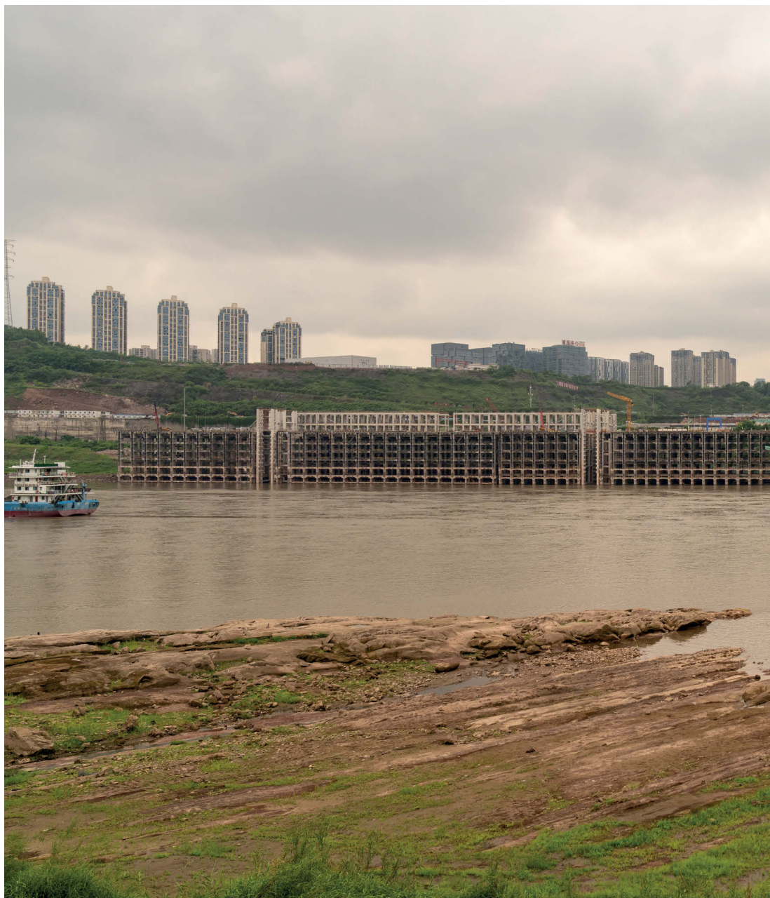
Concrete piers on the Yangtze river characterize the Lianglu-Cuntan Free-Trade Port Area in Chongqing, China.
