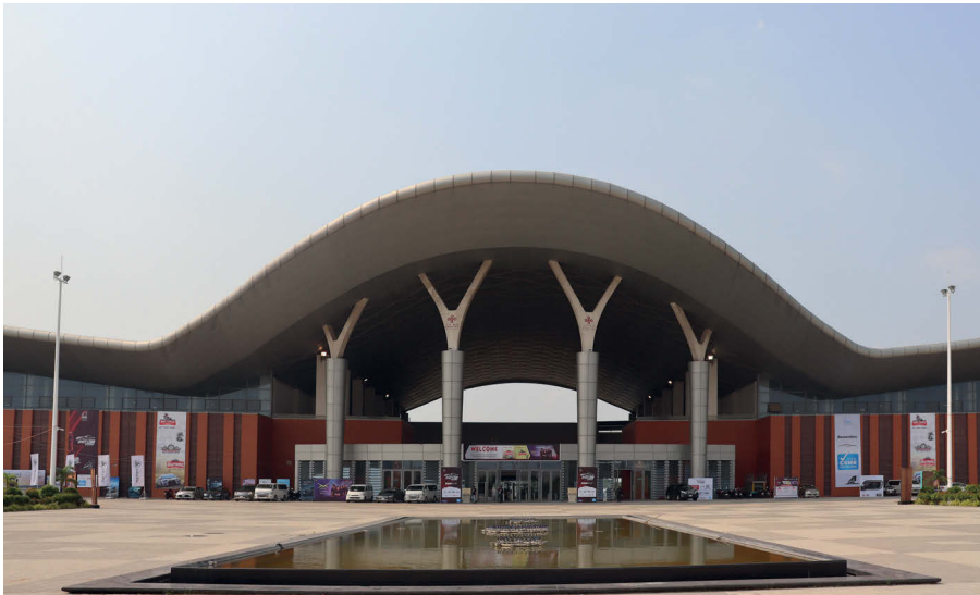
The façade made of red terracotta tiles is protected by a suspended big roof.
