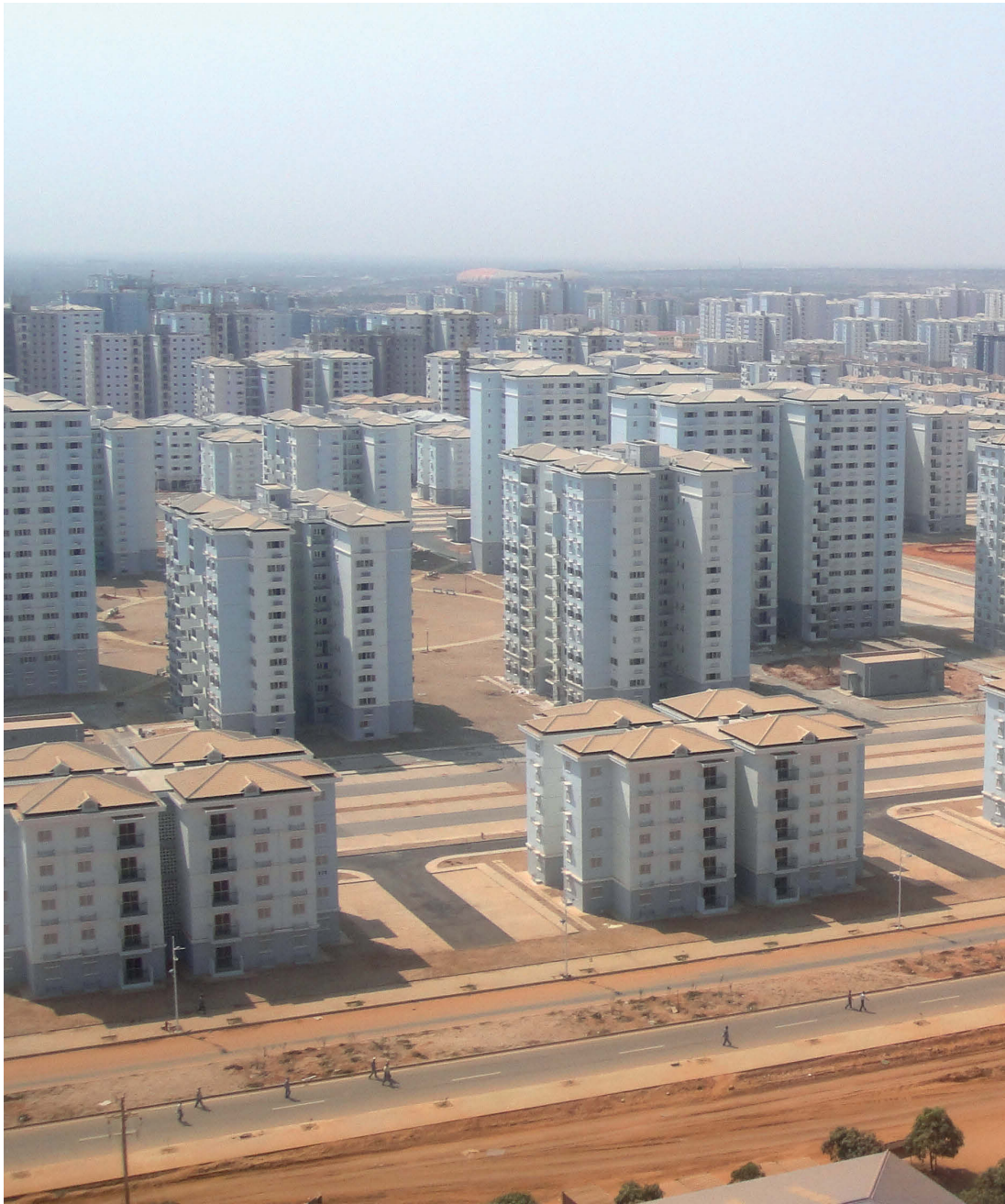
Repetition of mid-rise and high-rise buildings in Kilamba Kiaxi Housing Estate, Kilamba, Angola.
