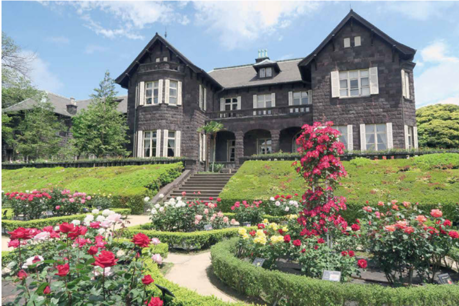
Figure 2.11. The main house, designed by Josiah Conder, overlooks the garden of the former Furukawa estate. Photograph by the Kikuchi Masayoshi.
