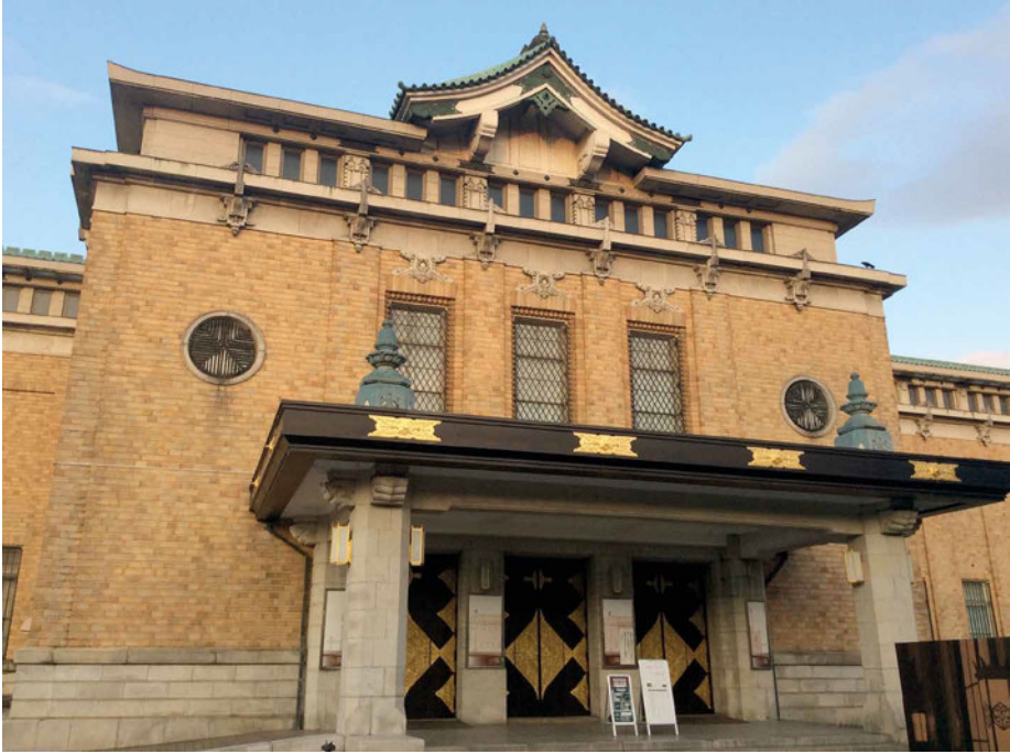
Figure 2.5. The entrance of the Kyoto Municipal Museum of Art (now the Kyoto City KYOCERA Museum of Art) references various historical styles but is modern in function. Photograph by the author.
