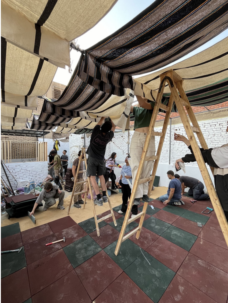
Figure 23: Winter School Building Resilient Cities, Cairo, 2024. Source: Juliana Canedo
