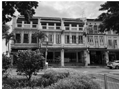
Figure 11.1b Shophouses in Singapore.
