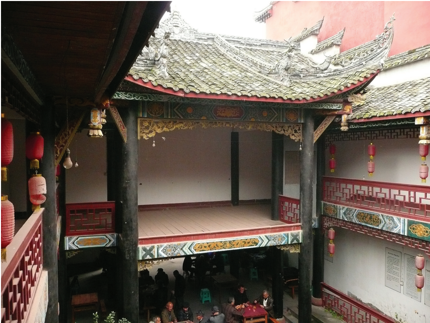
PLATE 14 Theater stage of the Bao lineage temple 包氏祠堂 in Longxing Town. The structure was reconstructed in the post-Mao decades. COURTESY OF THE AUTHOR
