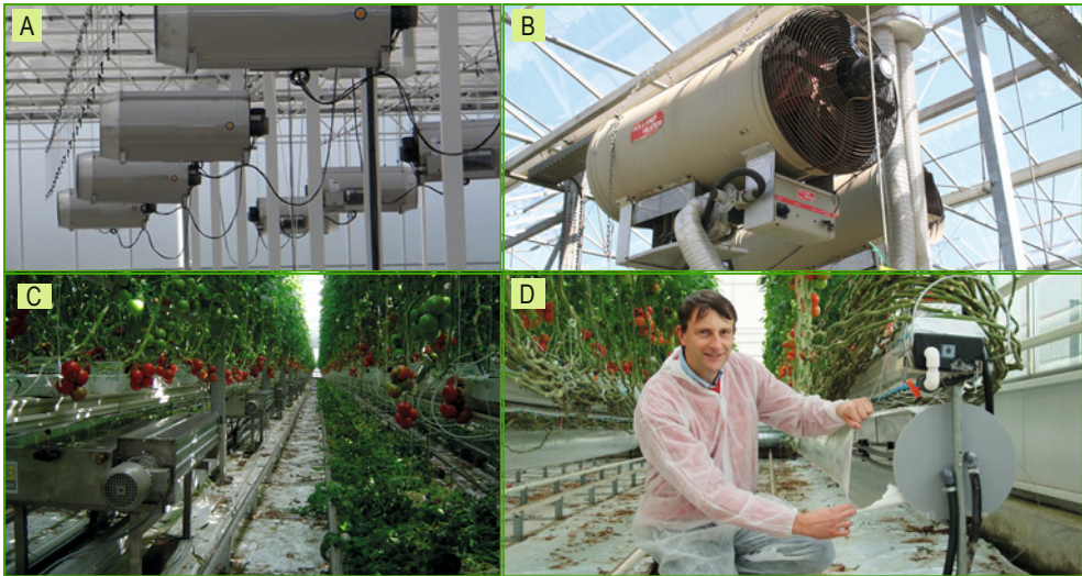
Figure 8.4. Direct heating systems where a fuel is burnt in a flame chamber and flue gases are added directly to greenhouse air (A) and an indirect heater (B) where fuel is burnt inside but flue gases are dispersed in outside air. ( https://www.winterwarm.nl/producten/agri/dxadxb_heater.aspx ; www.gvzglasshouses.co.uk ). Convective heaters, Fiwihex heat exchangers ( https://www.fiwihex.nl ) (C), and perforated tubes with water filled heating tubes or pipes (D).
