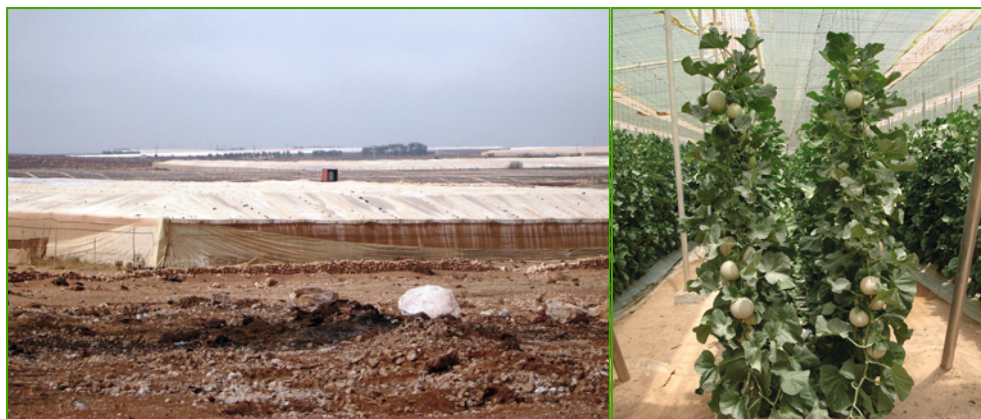
Figure 12.1. Left: 'Canarian' greenhouses in Morocco. The cover are two iron nets enclosing plastic (usually polyethylene) sheets separated by a 'ventilation' gap, fitted with a net against insects. Side wall ventilation is ensured by pulling down the lateral sheets, the opening fitted as well by insect screens. All gaps can be manually adjusted. Right is an inside view of such a greenhouse, with a melon crop (photos: Paolo Battistel, Ceres s.r.l.).
