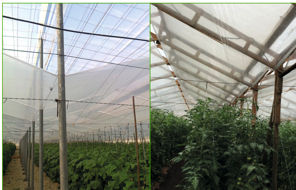
Figure 6.2. Transparent film placed below the greenhouse cover in the cold months, both to collect dripping condensed water and to increase insulation. Left, in a parral greenhouse with cucumber, in Almeria and right, a wooden greenhouse with tomato near Valparaiso (Chile). (photos: Cecilia Stanghellini)
