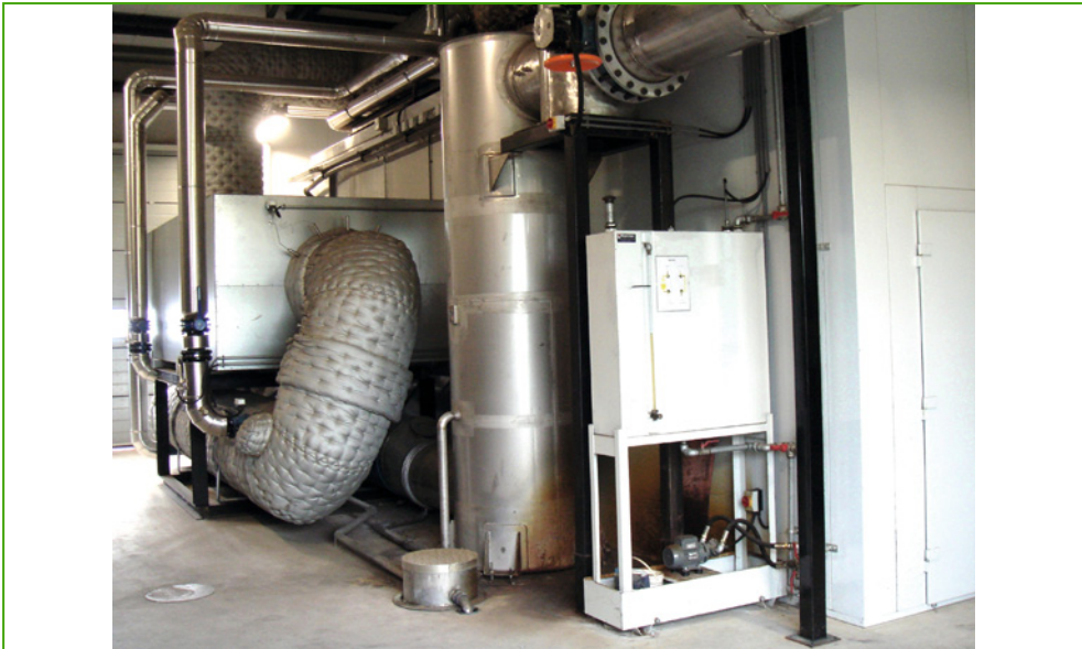
Figure 11.1. Example of technology required to make exhaust gas of a combined heat and power (CHP) motor suitable for CO 2 enrichment in a greenhouse (see also Figure 8.10). The motor is behind the sound-insulating white wall and liquid urea is sprayed into the exhaust which has a temperature around 120 °C. What we see here is the cooler: the thick insulated duct comes from the motor (up, left, in the back) enters the cooler (centre, left) and is sent to the greenhouse (up right), after that water is condensed and recovered in the pit (centre, bottom) (photo: Paolo Battistel, Ceres s.r.l.).
