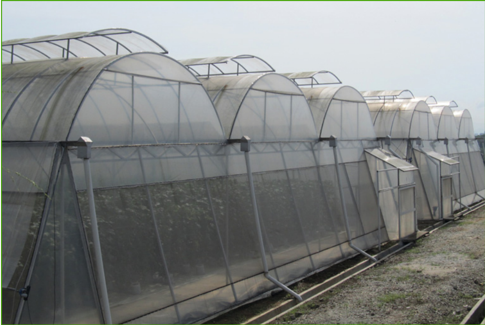
Figure 5.1. Greenhouses in tropical low land (near Kuala Lumpur, Malaysia), designed (Campen, 2005) to take advantage of buoyancy in the absence of wind (photo: Anne Elings, Greenhouse Horticulture, Wageningen University & Research).
