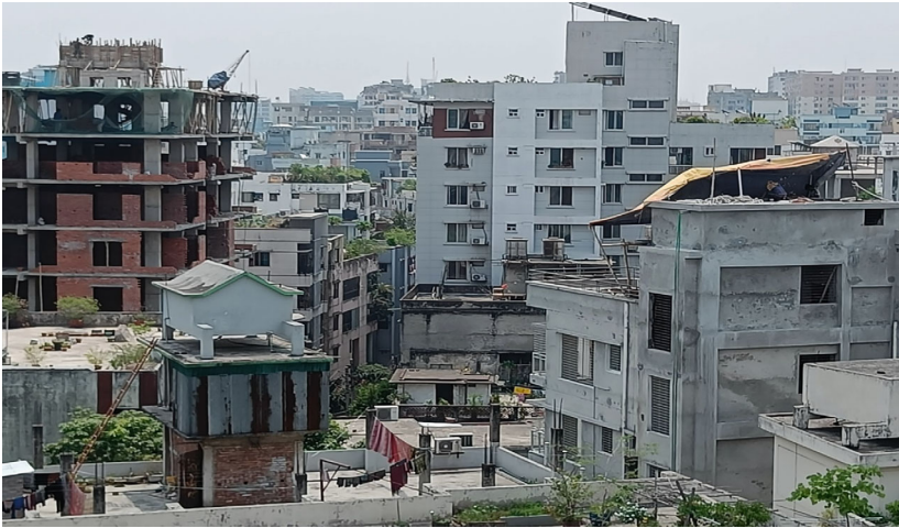
Fig. 3.3 Selective housing redevelopment in Dhaka City. Photo by Ya Ping Wang
