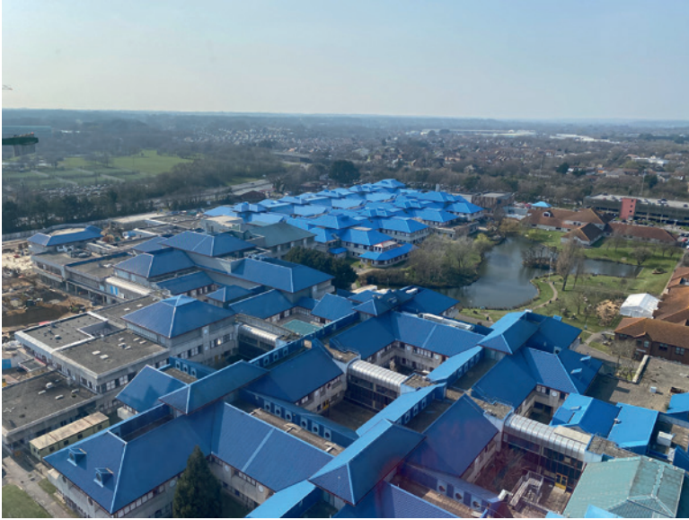
Figure 5.4 The blue roof of Royal Bournemouth General Hospital.
