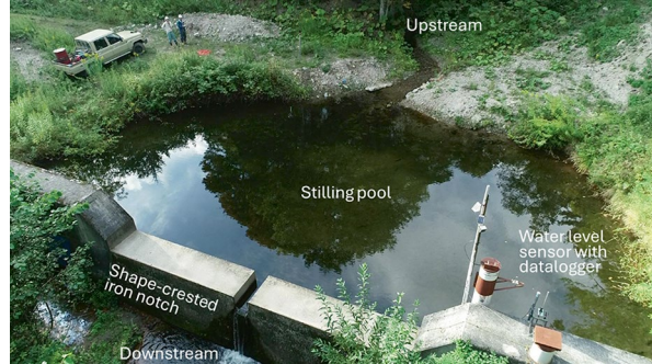
Fig. 4.4 Bird-eye view of Maruyamasawa streamflow gauging station. (Photo by the UTHF, licensed under CC BY-NC-ND 4.0)
