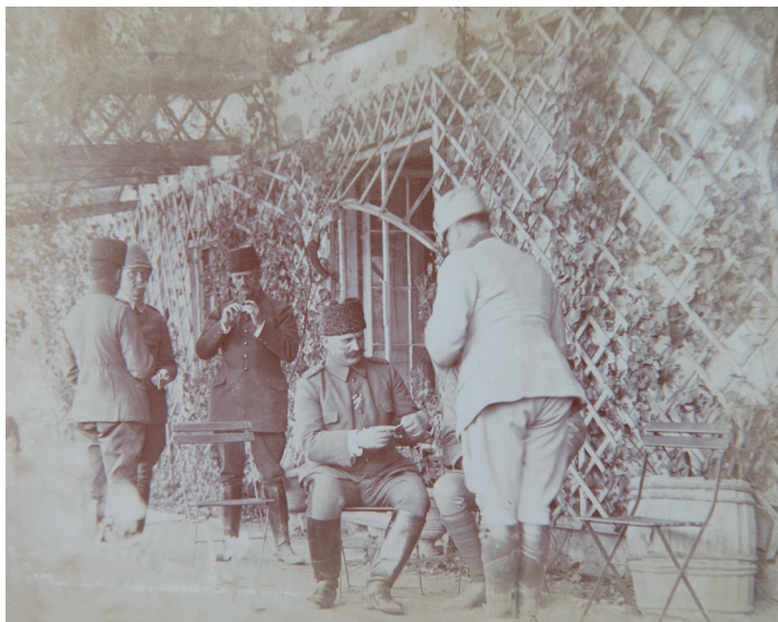
Figure 37 Thymbra Farm served as military quarters for the Ottomans during the Battle of Gallipoli in 1915/1916
