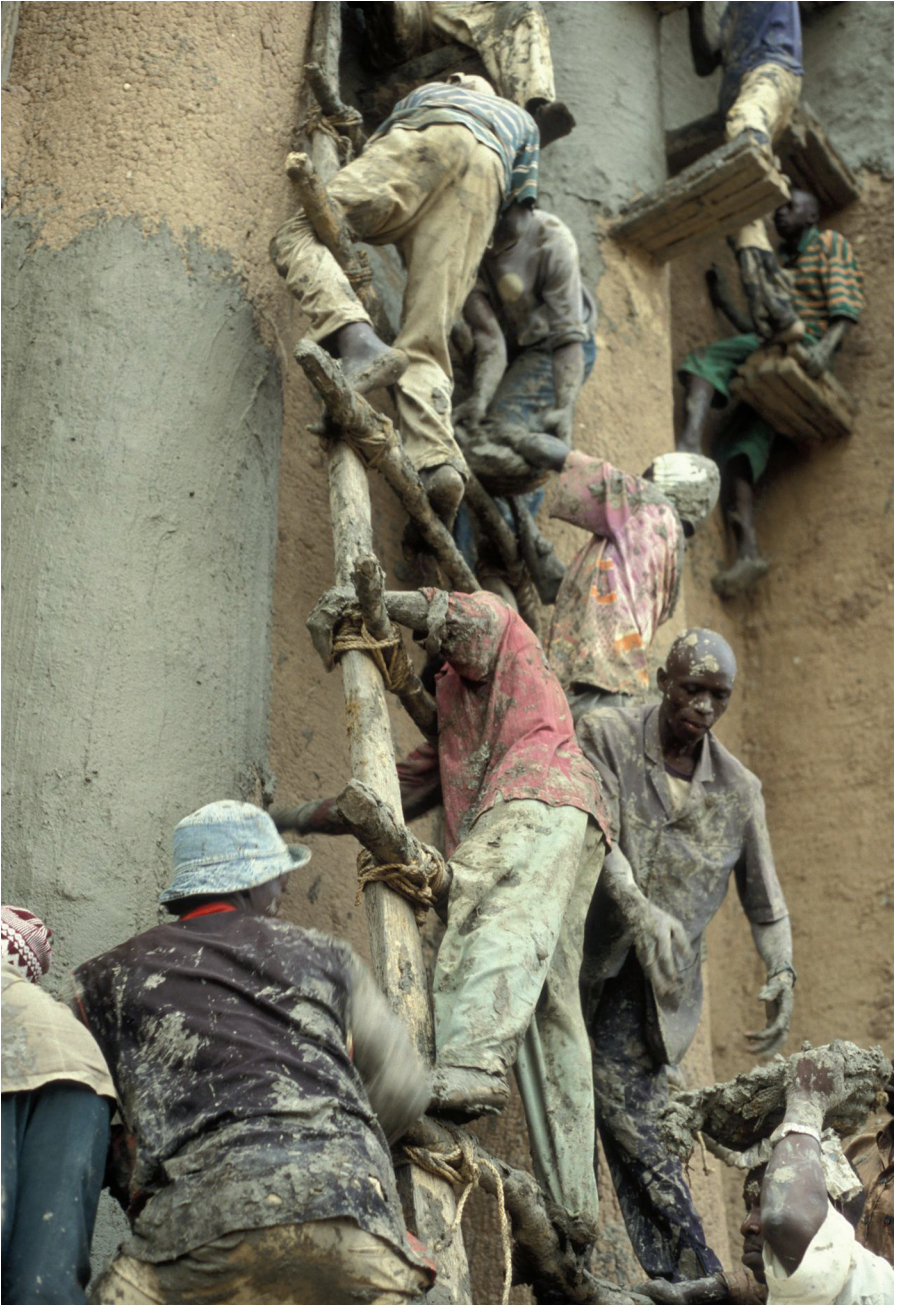
Plate 14 Re-claying the Djenné Mosque
