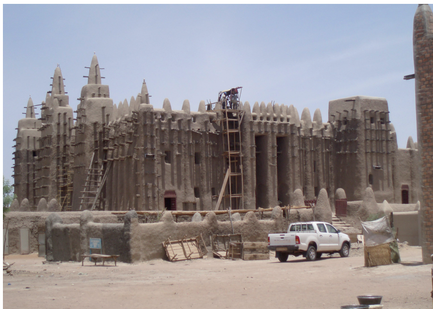
Plate 15 An early stage in the AKTC restoration works
