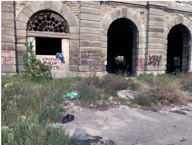
Fig. 2: The occupied Silos in 2024
