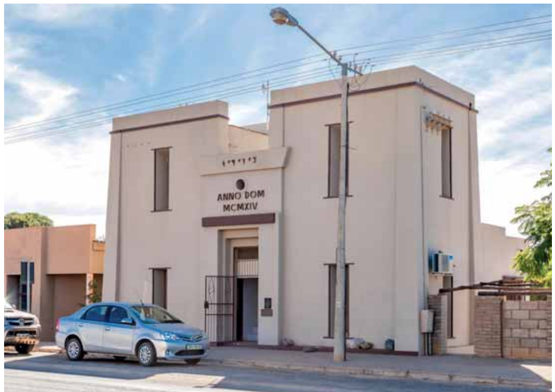
Figure 44: A.B. Hangartner. Transformer building, Kakamas. 1914 (photo courtesy of ID 160520746 © dpreezg, deposit-photos.com)
