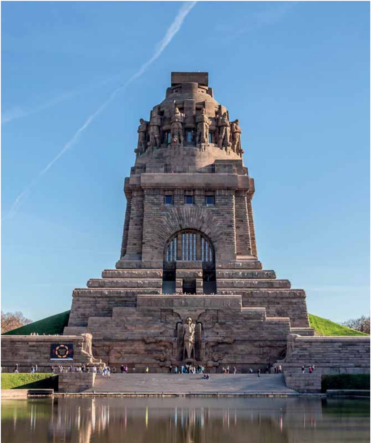
Figure 76: Bruno Schmitz et al. Völkerschlachtdenkmal, Leipzig. 1913. Steel and concrete with granite facing, h. 91 m, plinth 70 × 80 m (photo courtesy of Alamy G0GD80)
