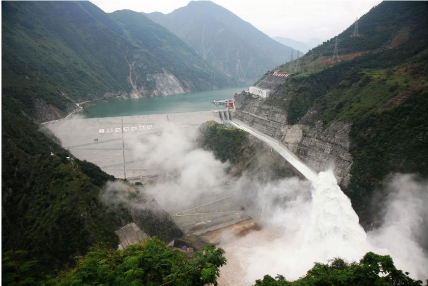
Fig. 1.8 Pubugou hydropower station
