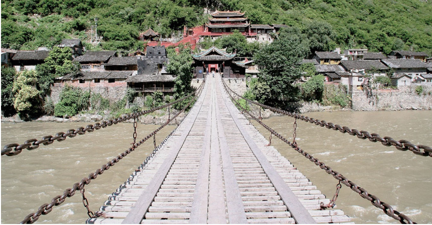
Fig. 1.6 The chain spans of the Luding Bridge
