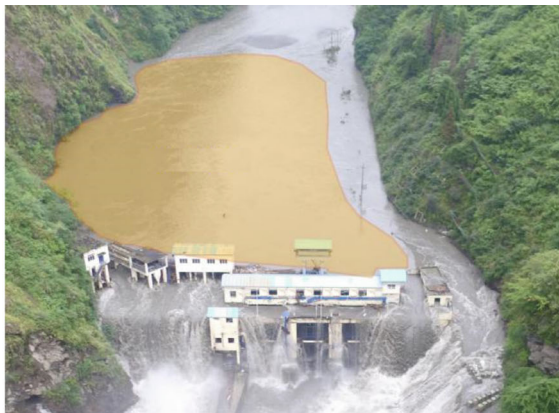
Fig. 7.7 Dam forebay area underwater measuring via USV-carried depth sounder
