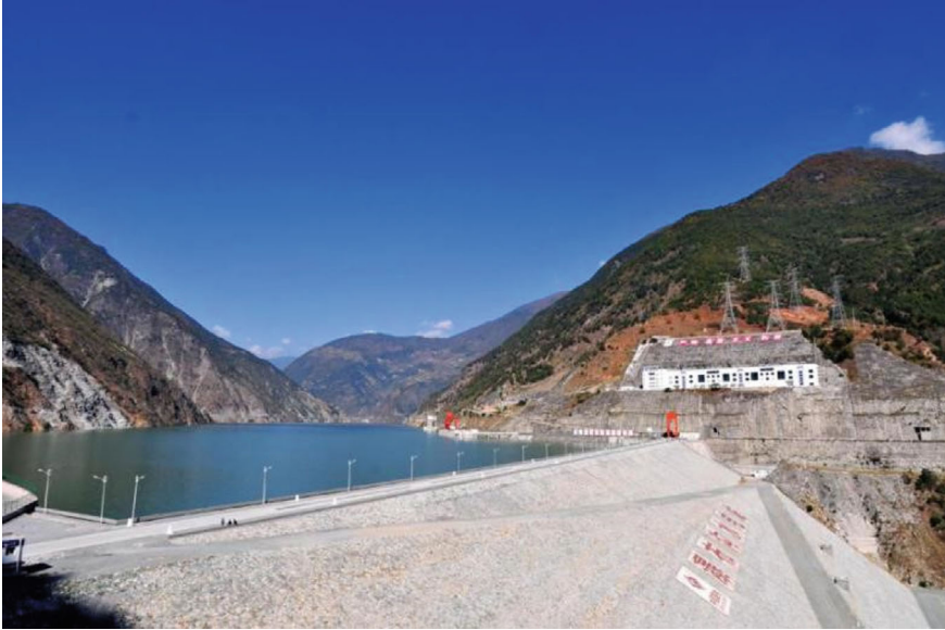
Fig. 2.3 International Milestone Project: The 186 m tall Pubugou gravel-soil core rockfill dam
