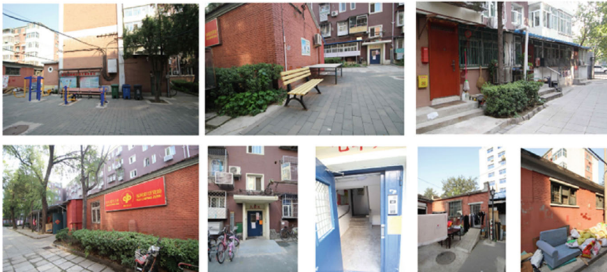
Fig. 16.1 Renovation in process in Daliushu Community, Beijing (Source Youyang Zhao)
