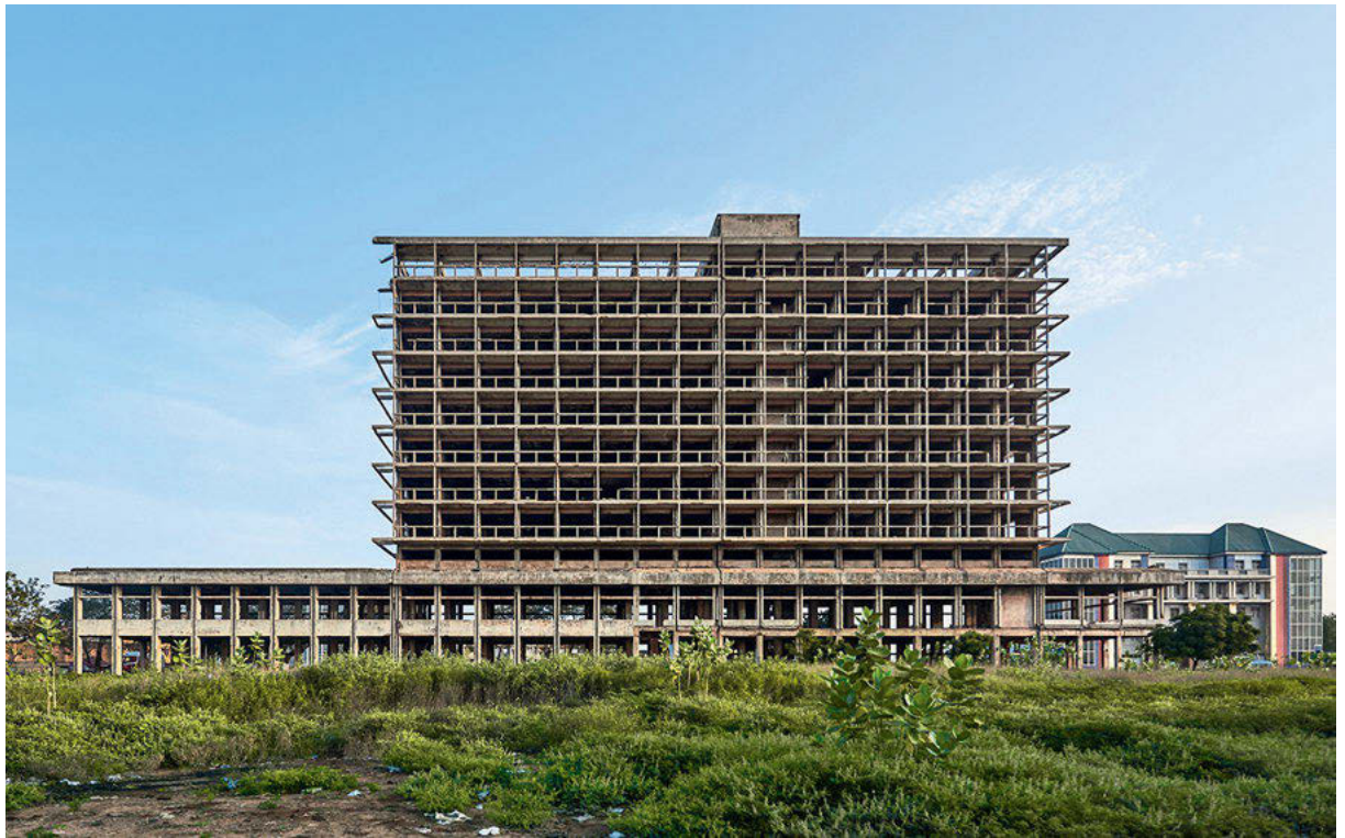
▲ The front view shows the cantilevered concrete beams with embedded brise-soleils.
