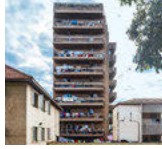
Mary Stuart Hall of Residence Extension (1972), Uganda
