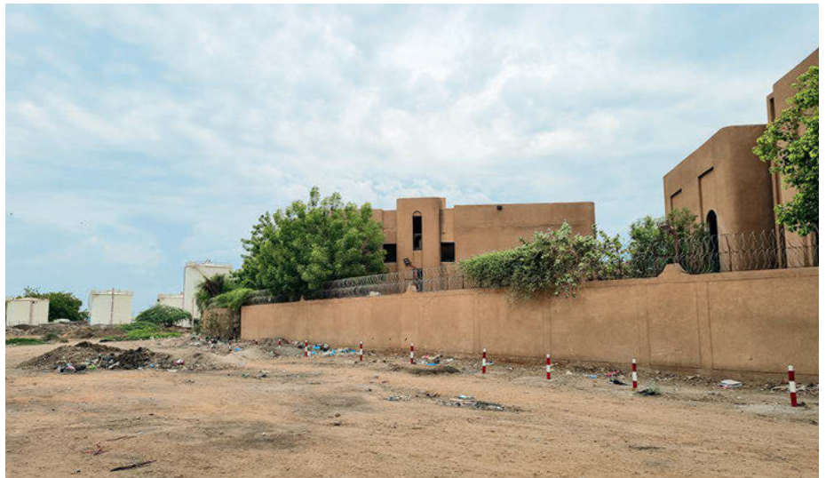
▲ View of the enclosed complex.
