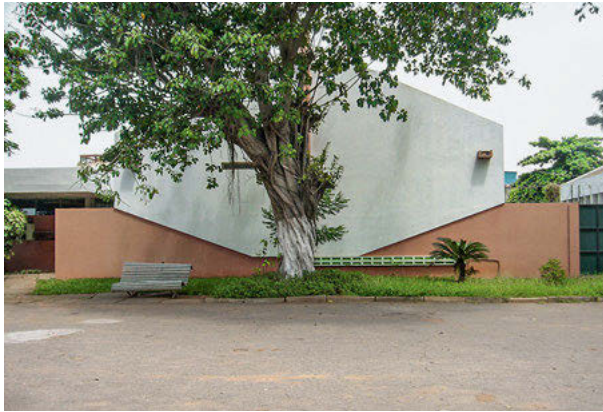
▲ Gable wall of laboratory.
