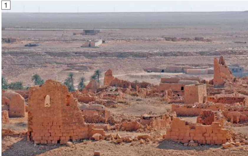
Fig. 6.9. (left) Myd(---)/Gheriat el-Garbia, north-western Libya: main gate ( porta praetoria ) of Severan fort. 1: Gate towers with collapsed outer central arch, with Berber village in the fort's interior; 2: Excavations between the gate towers seen from the interior of the fort (photos M. Mackensen).
