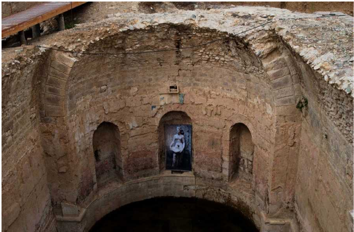
Figure 3. The Northern Thermal Spring of Allianoi - Apsidal Section in the North of A1 Hall (Photo M. Günör)
