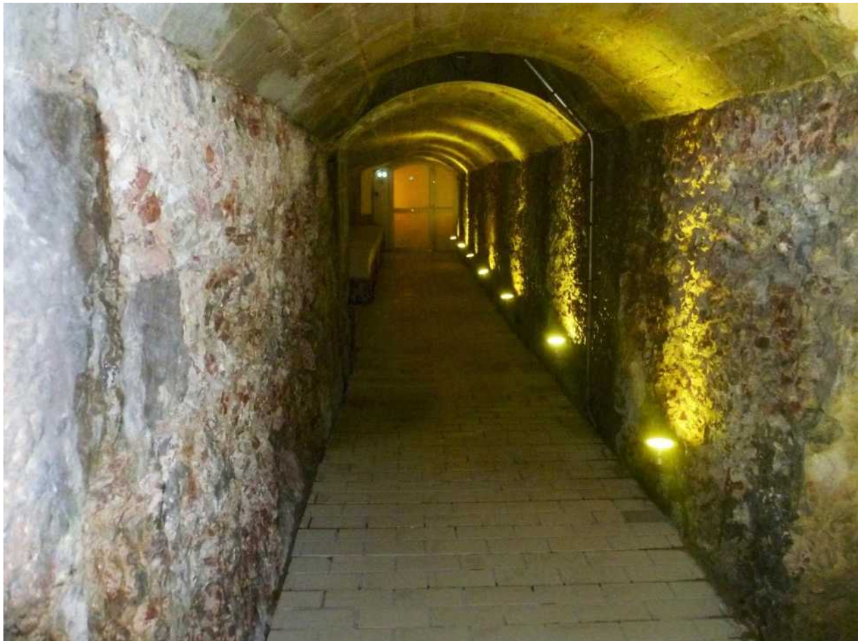
Figure 6b. Photo of the Jutier corridor in Plombières-les-Bains, excavated in the Roman opus caementicium slab (photo by https://remiremontvallees.com/2019/06/12/plombieres-les-bains-et-ses-vestiges-antiques/ , viewed 12 th June 2019).
