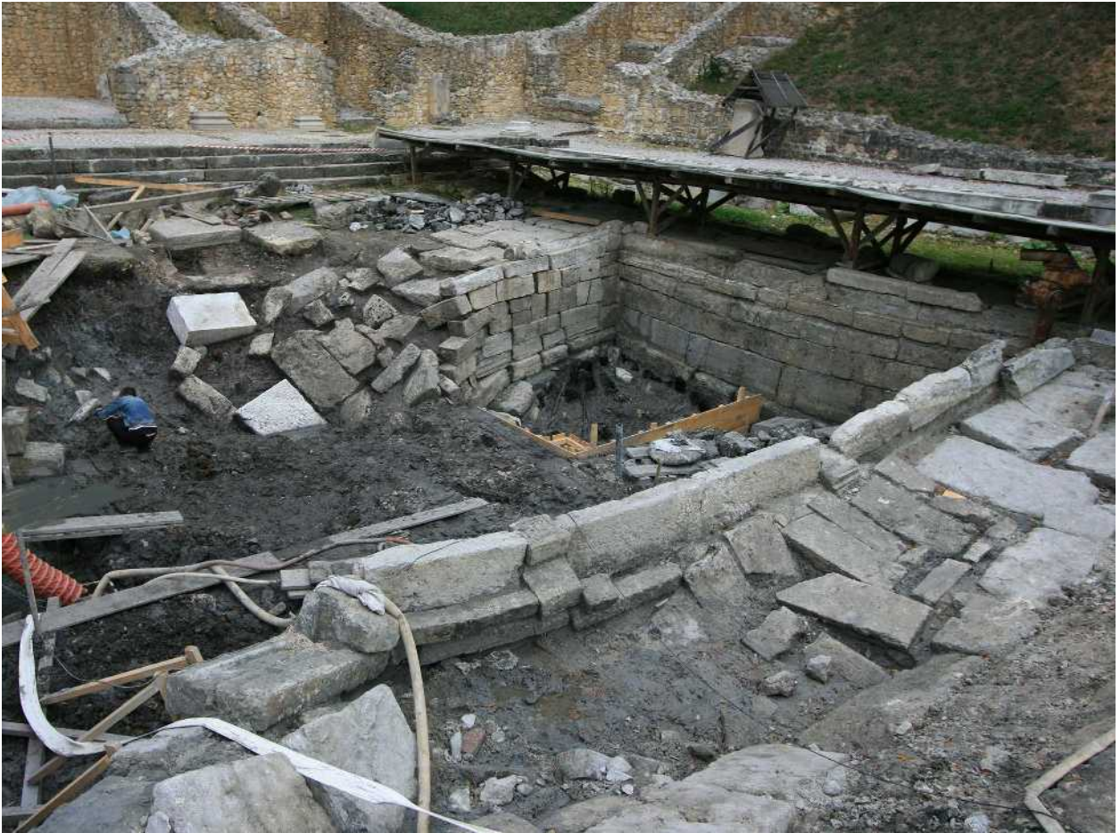
Figure 3. Roman spring reservoir during the 2011 excavations looking north-east ( photo by D. Nemeth-Ehrlich).
