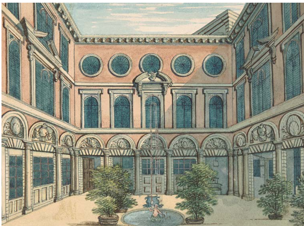
Figure 126 The courtyard of Tallow Chandlers' Hall by Samuel Ireland, between 1794 and 1800 (Yale Center for British Art, Paul Mellon Collection, B1977.14.9480). The hall was built in 1671–3 by the master bricklayer Captain John Caine, and is very like Brewers' Hall in Addle Street which he also built (destroyed in World War II)
