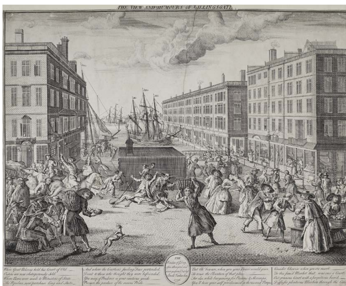
Figure 20 Billingsgate dock from the north in 1736 by Arnold Vanhaeck (LMA, London Picture Archive 319833; this version of 1762). There is no information on the dark-shaded building in the centre of the picture. The way through to Smart's Key can be seen at the far end of Beckford's house, on the left (compare Figure 19)
