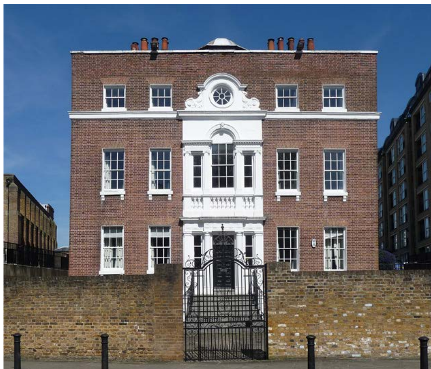
Figure 135 Nelson Dock House, Rotherhithe (Stephen Richards, Wikipedia Creative Commons). The belvedere is the cone-shaped roof between the chimney stacks
