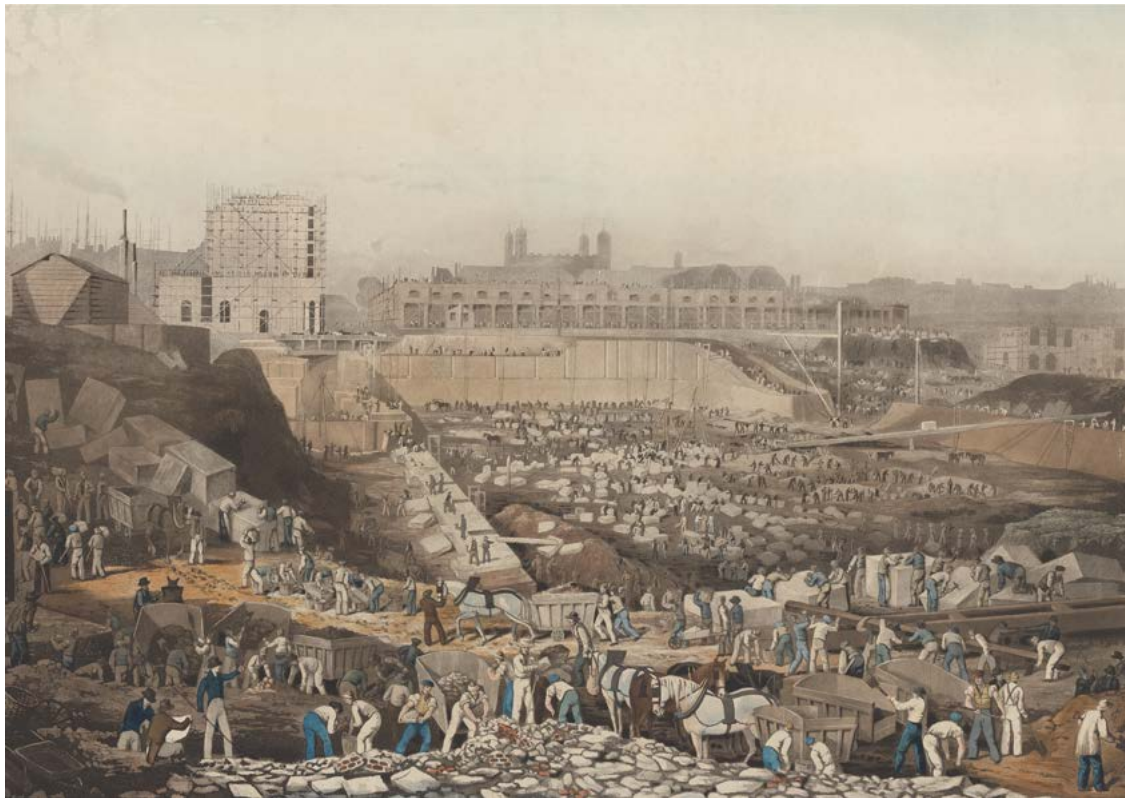
Figure 191 Excavation for St Katharine's Docks in progress, 1828, by an unknown artist (Yale Center for British Art, Paul Mellon Collection, B1977.14.12781). The view looks west towards the Tower
