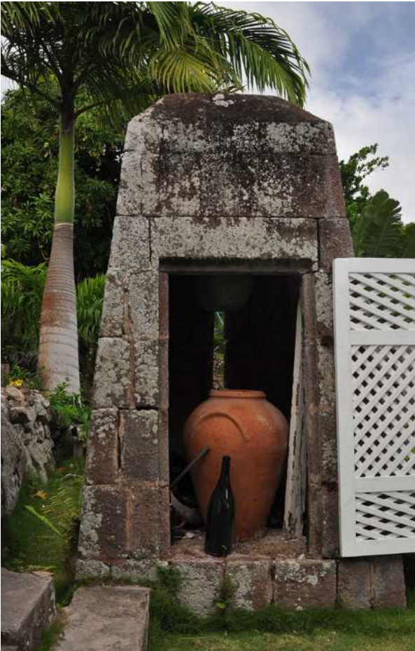
Figure 1.11. Hermitage: drip filter with reused 18th-century Montelupo olive oil jar inside to catch water (photograph: Robert Philpott, 2013)
