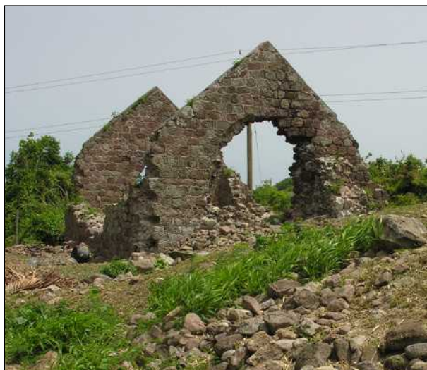
Figure 2.9. Fenton Hill: boiling house (B) from N
