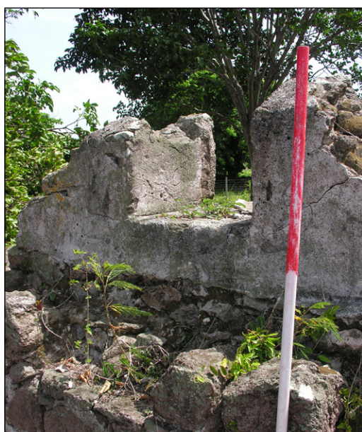
Figure 2.18. Fenton Hill: Structure A, E wall from outside showing window in gable and offset wall for gutter
