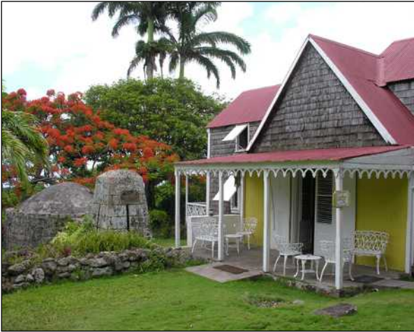
Figure 2.41. Hermitage, Nevis: late 17th-century estate house showing shingled exterior; the domed cistern and drip filter stand to left of main house
