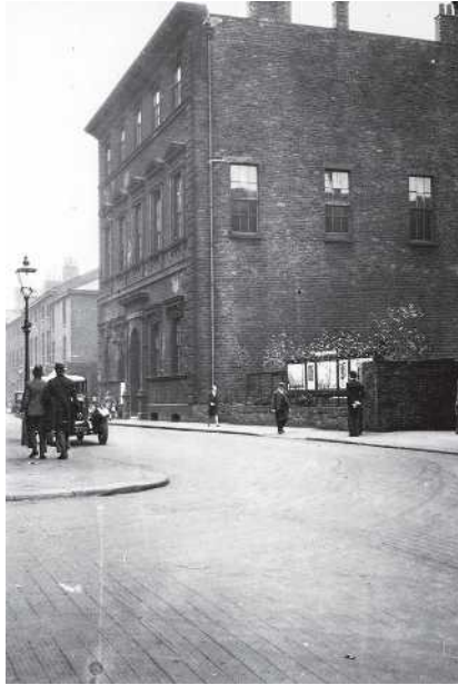
Figure 101 Photograph of Mechanics Institute, Surrey Street, Sheffield, England. (Picture Sheffield, Reference: s06452. Sheffield Archives and Sheffield Local Studies Library.)
