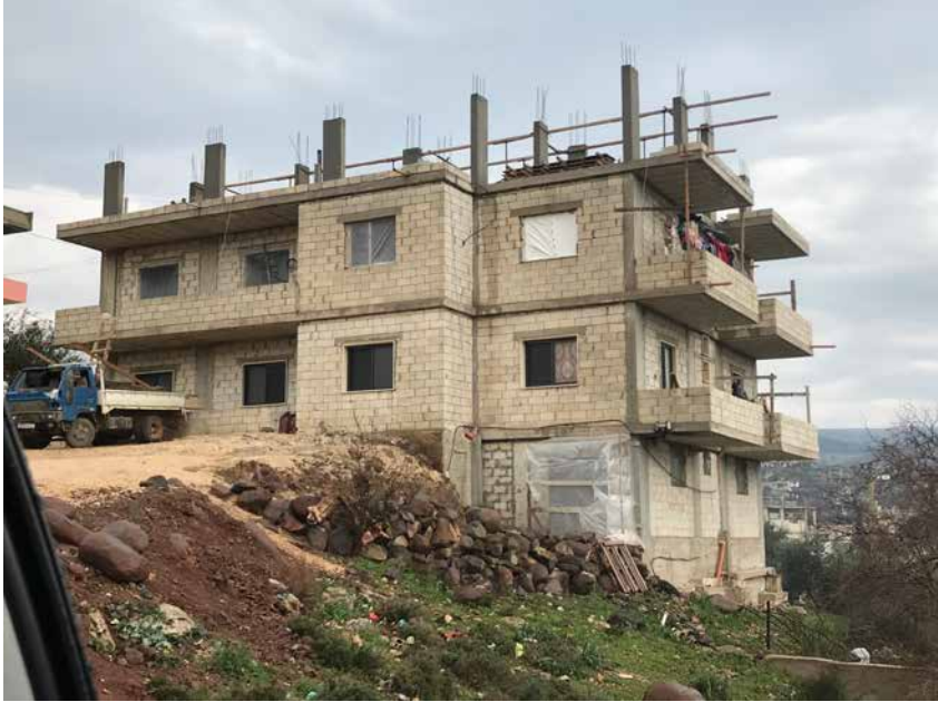
Figure 6.1. OFC building in Amayer. © Watfa Najdi.
