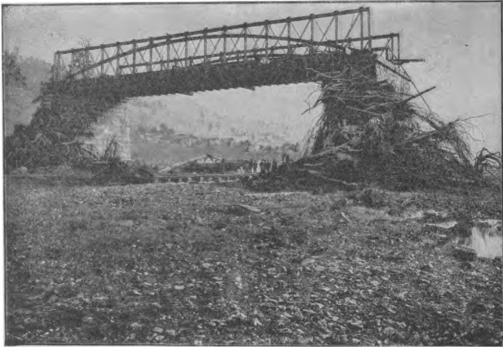
THE SPAN OF THE WOODVALE BRIDGE THAT WITHSTOOD THE FLOOD.
