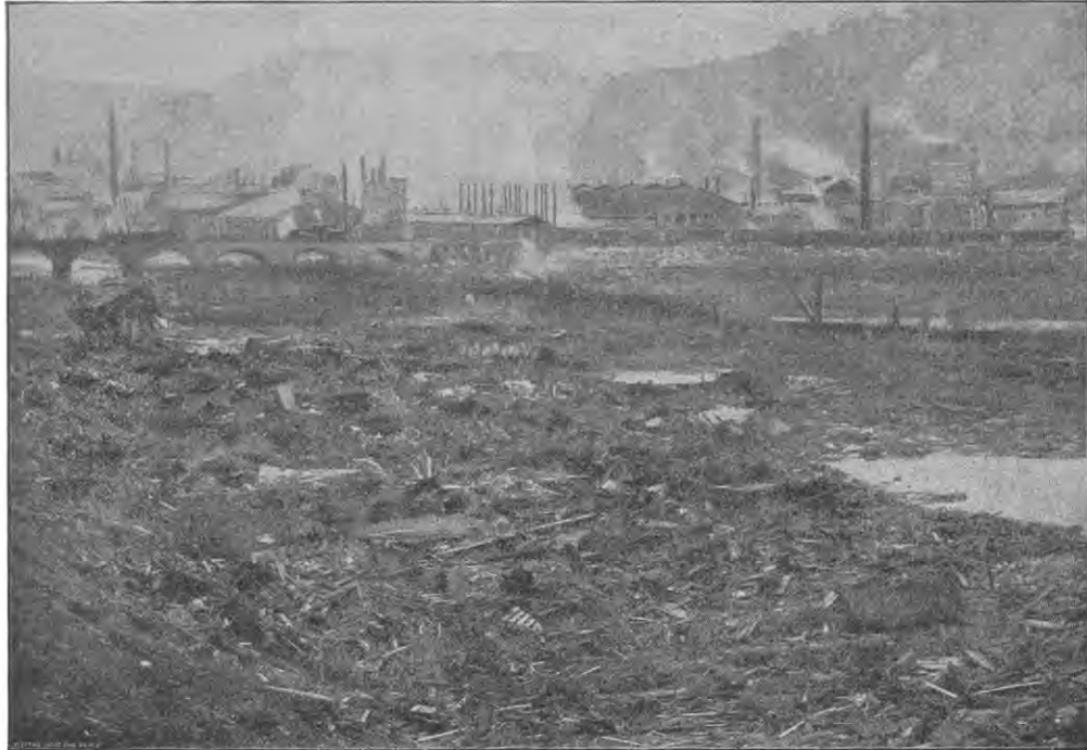
ABOVE THE RAILROAD BRIDGE AND CAMERIA IRON WORKS TEN DAYS AFTER THE FLOOD
