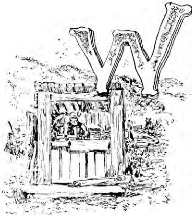
FIRST BUILDING AFTER THE FLOOD.
