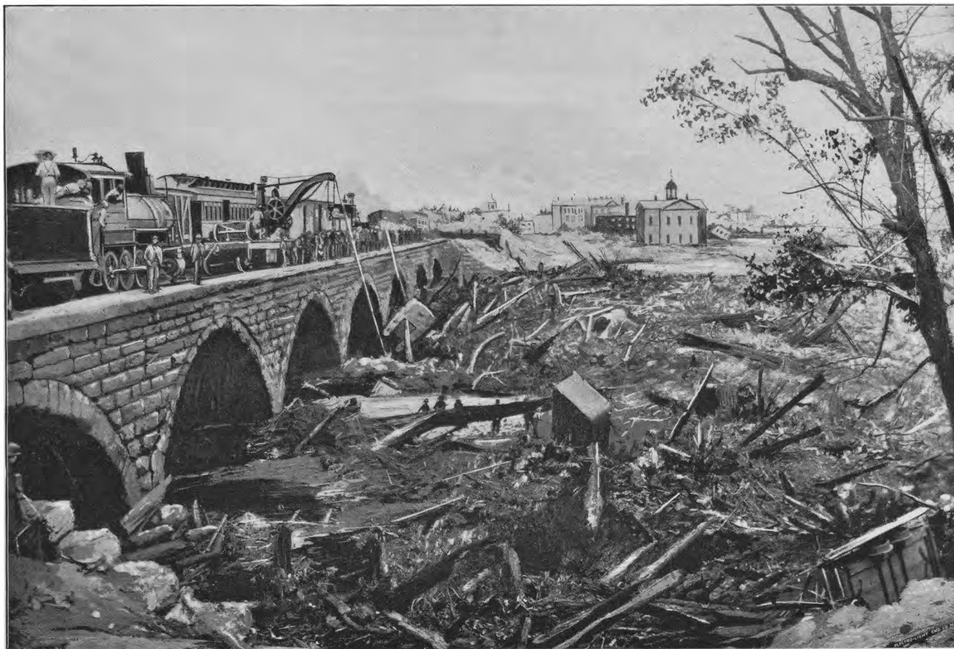
WRECKING CAR CLEARING AWAY THE DEBRIS ABOVE THE STONE BRIDGE.
