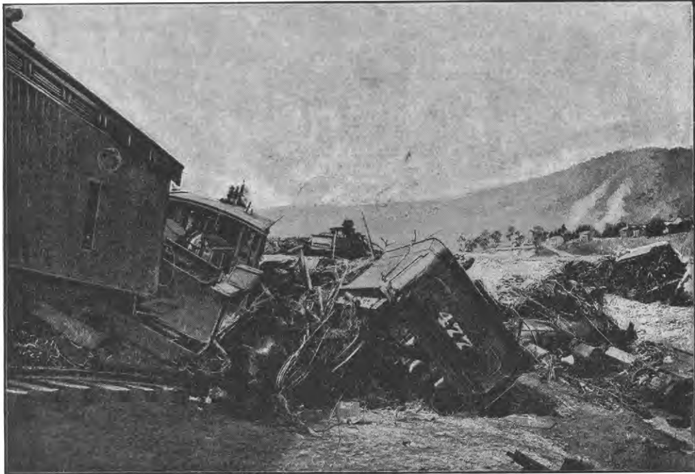
RAILROAD WRECKAGE AT EAST CONEMAUGH.
