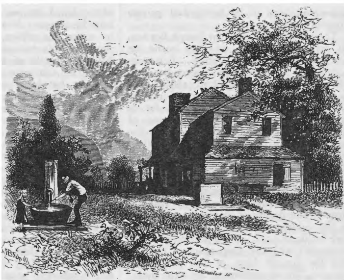
OLD HOUSE AT JAMESBURG.
