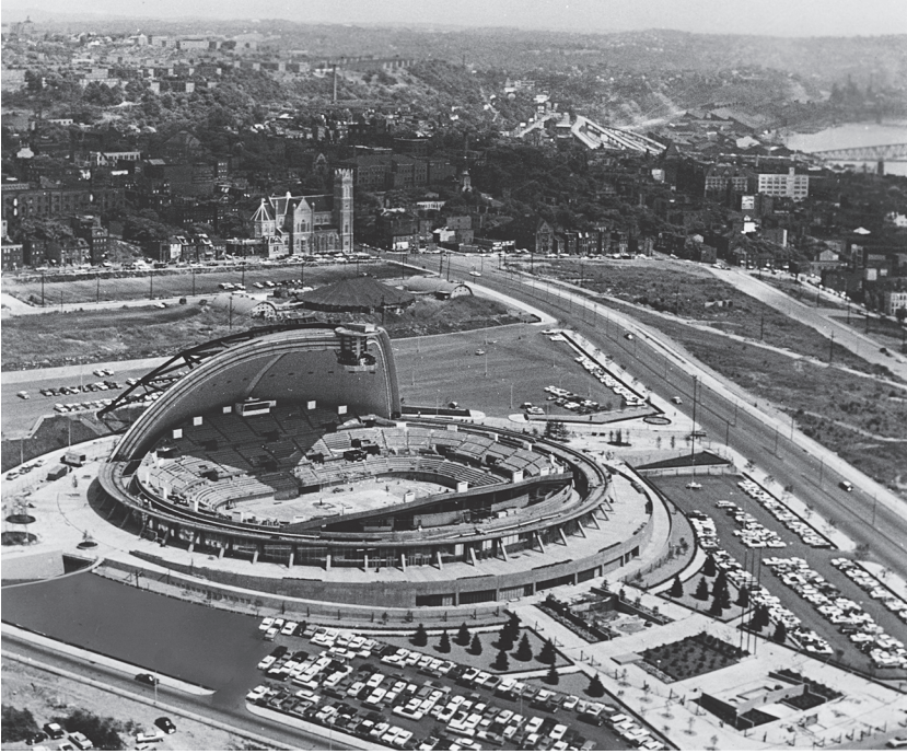
Fig. 5. View of the Civic Arena in the Lower Hill, Pittsburgh. Freedom Corner is to the right of the church at the center top of the photo. Photograph by Robert E. Dick. Allegheny Conference for Community Development, Detre Library & Archives, Senator John Heinz History Center, Pittsburgh, PA. Image courtesy of dck Worldwide Group, LLC.
