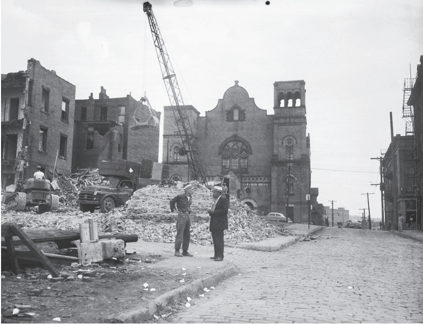
Fig. 3. Demolition zone for the Civic Arena, with Marpec Construction Company Contract Hauling truck, in front of Bethel AME Church, possibly Elm Street, Lower Hill District, in Pittsburgh, 1957. Photograph by Charles “Teenie” Harris (American, 1908–1998). Black and white, Kodak safety film, 4 × 5 in. (10.20 × 12.70 cm). Carnegie Museum of Art, Pittsburgh. Heinz Family Fund, 2001.35.4091. Photograph © Carnegie Museum of Art, Pittsburgh.
