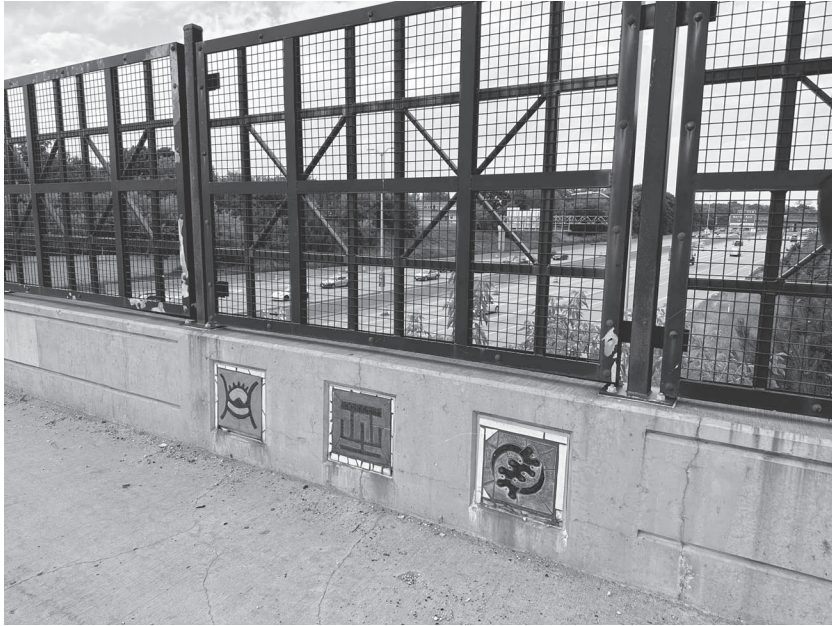
Fig. 15. Walnut Street Bridge, Milwaukee. Photo: author
