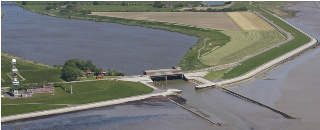
Figure 1: Tide gate and pumping station Knock in the area of the water board Emden at the East Frisian coast (Source: I. Entwässerungsverband Emden).
