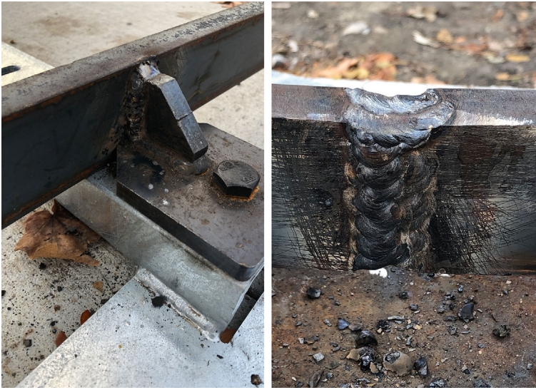
Fig. 6.5 A bracket on the new pedal-car rails (left) and my double V-groove splice that wasn't straight (right)
