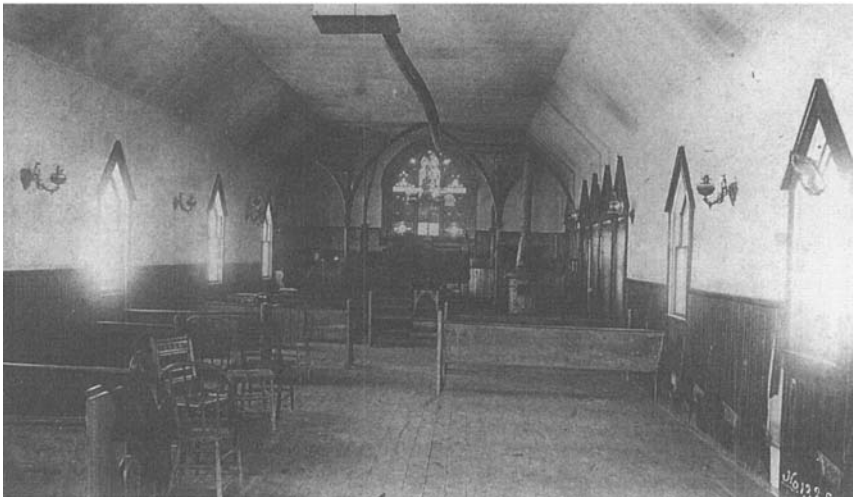
Interior of the Episcopal Church after all of the wounded Lakota were removed. Photograph by Clarence G. Morledge, courtesy of Rohan Collection, Nebraska State Historical Society.
