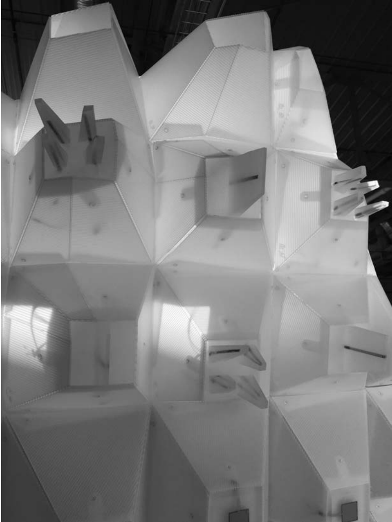
FIGURE 11.94 Silicone controllers in place within the waffle frame wall system
