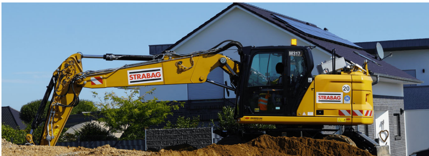
Fig. 1 Excavator used for field study
