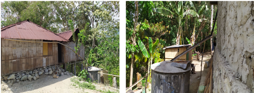
Fig. 8.6 Innovative housing design in Nangapanda featuring integrated rainwater reservoirs
