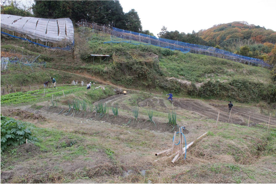
Fig. 2.4 Completion of farmland recovery at the project site
