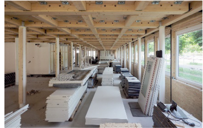
Fig. 6. Disassembly process (Lukas Lang Building Technologies).
