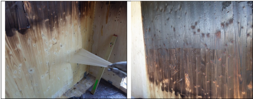
Fig. 8. Left: Removal of dried soot removal film; Right: Cleaned and uncleaned surfaces.
