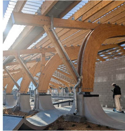
Fig. 4. Reused glulam in forefront, new glulam arches in the back by Esther Vandamme.
