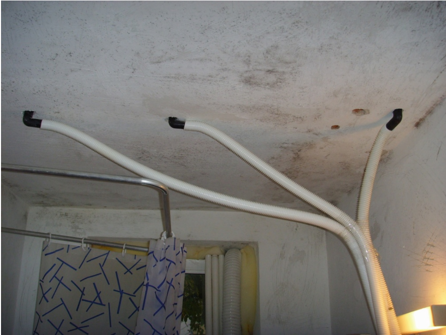
Fig. 3. Drying of wooden-beam ceiling with overpressure method
