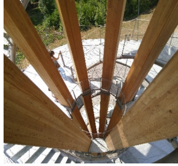
Fig. 1 Larch GL columns of the Schönbuchturm, Herrenberg, Germany.
