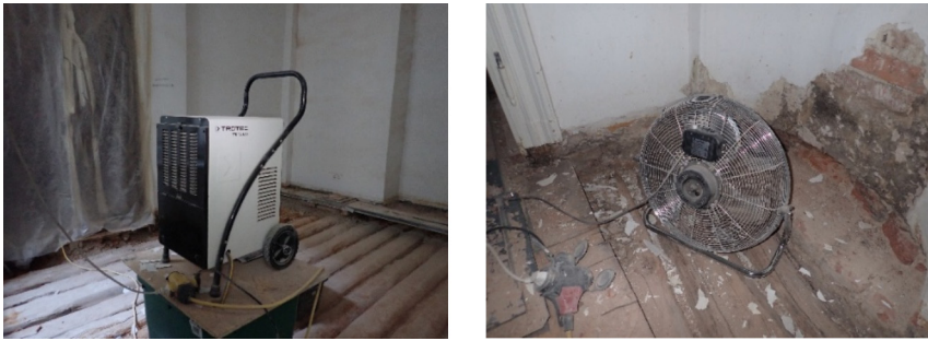
Fig. 1. Left: Condensation dryer; right: Ventilators help to guide the air flow during drying
