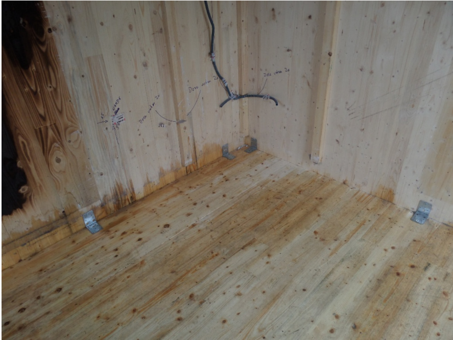
Fig. 4. Mass timber elements before drying; all panels were removed and the CLT elements were exposed
