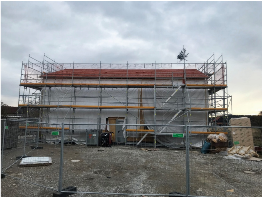
Fig. 6 Temporary sheeted weather protection to timber structure
