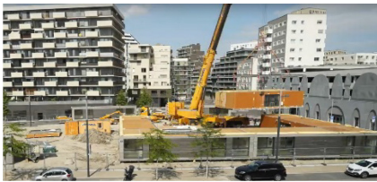
Fig. 7. Dismantling process (© Seestadt TV/Roland Thurner).
