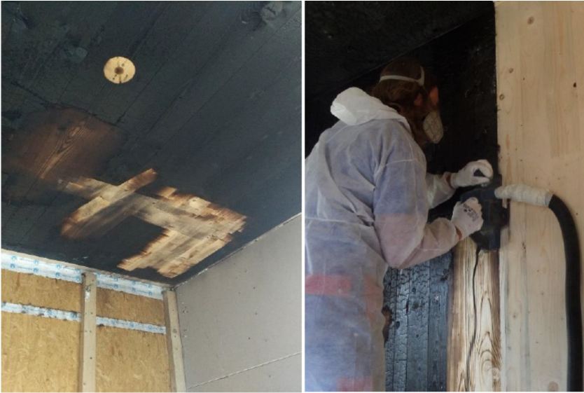
Fig. 9. Renovation of the wood surface using planing and sanding methods
