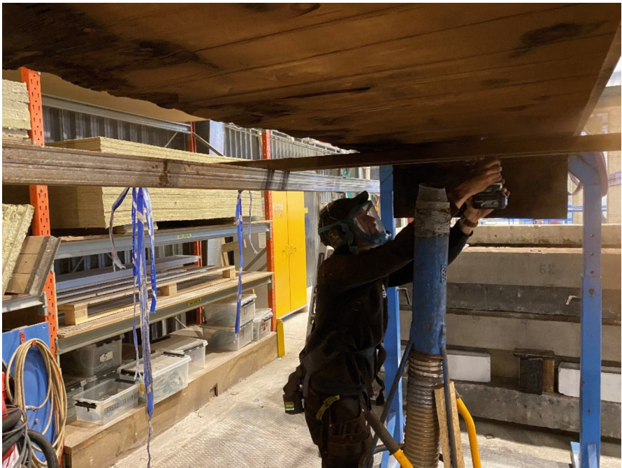
Fig. 11. Experimental setup for post-fire repair of a section of a compartment ceiling after a severe 4 h long fire [27]
