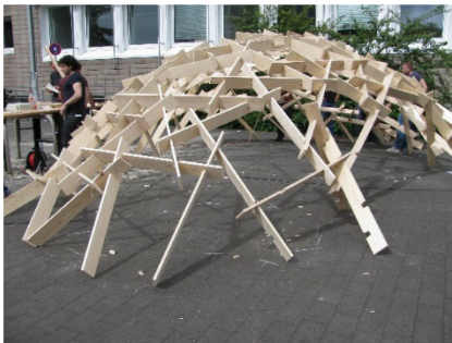
Fig. 1. Assembly of a reciprocal framework by Alec Singh.
