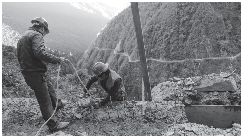
Figure 9: Construction work on the road between Gongshan and the Dulong Valley (picture by the author, 2016)
