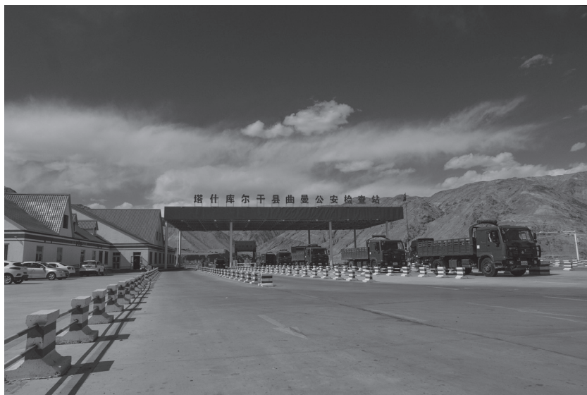
Figure 17: A new permanent checkpoint along the KKH near Tashkurgan (picture by the author, 2017)
