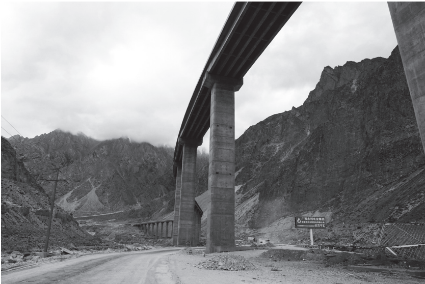
Figure 15: Suspension bridges on the new KKH in the Gez Canyon (picture by the author, 2016)
