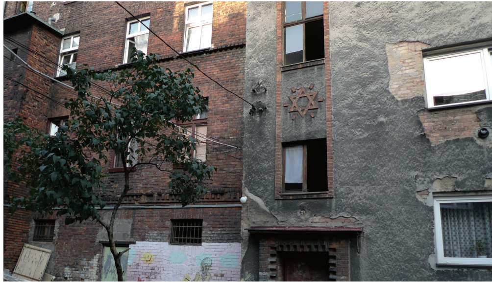
4.8 A courtyard in Bytom at 6 Smolonia Street, photograph by Natalia Romik.
