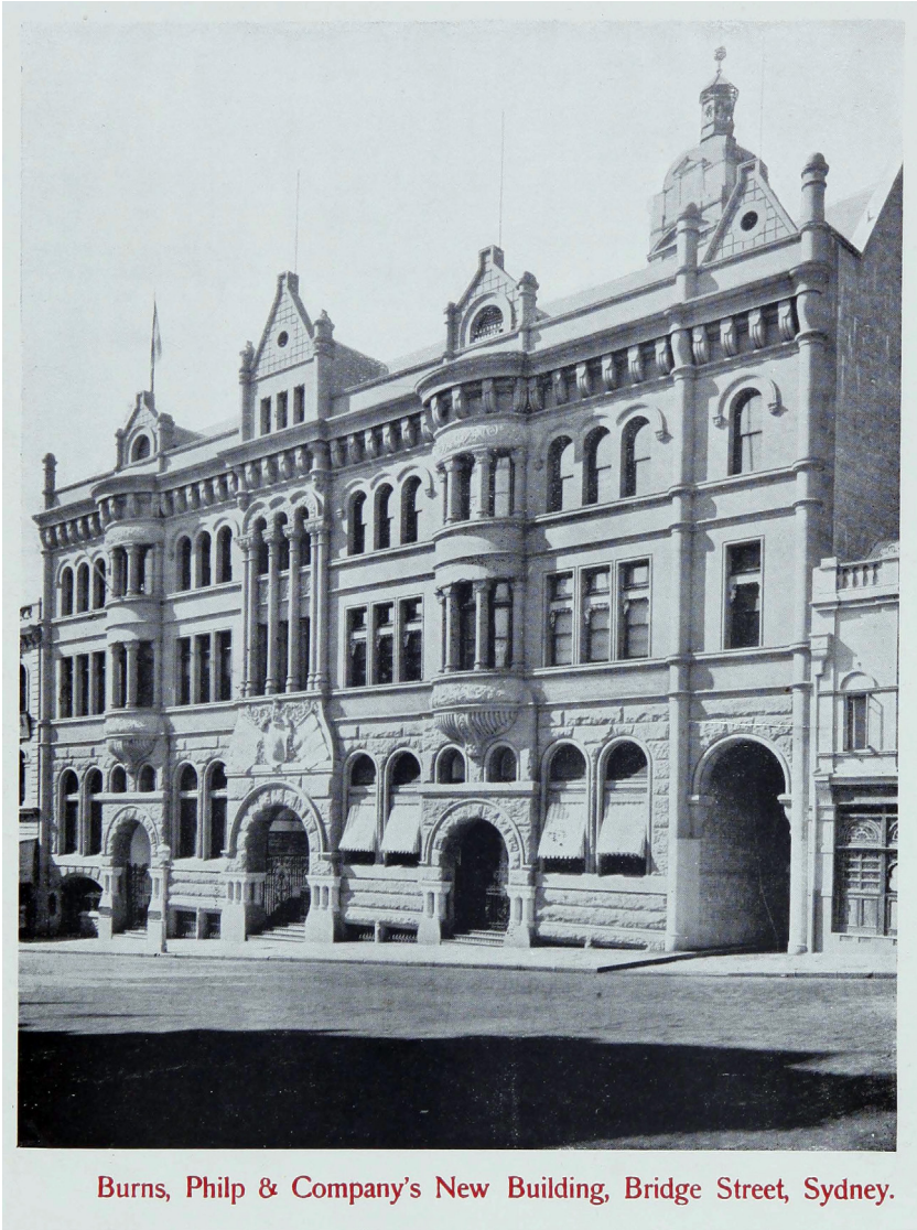
Fig. 8.1: Burns Philp headquarters building, Sydney (Burns Philp 1903, 13)
