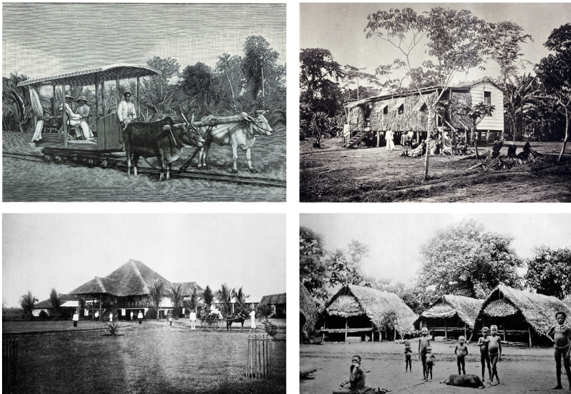
Fig. 7.3b–e: Features from Stephansort: (b) 'ox-train', (c) 'pharmacy', (d) 'administrative headquarter building of the Astrolabe-Compagnie' and (e) 'idyllic village of Bogadjim' (Hesse-Wartegg 1902, 61; Hagen 1899, pls. 6, 17, 37)
