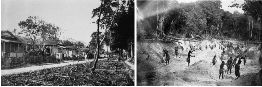
Fig. 5.6: (a) Prefabricated housing for the European employees of the German South Sea Phosphate Company in Angaur, supplied by F. H. Schmidt, c.1909; (b) Manual phosphate mining underway in the early period of the DSPAG's activities on Angaur. A tramway has been cleared through the old growth forest. Up to five metres of phosphate have already been removed in some areas, c.1909 (Deutsches Bundesarchiv, Sammlung Heinrich Hagedorn, Bild 223–158 and 223–153)
