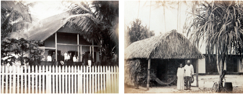
Fig. 4.3 a–b: The different appearances of the houses in Knappe’s photograph album allow conclusions to be drawn about the financial means of the local entrepreneurs and settlers (private collection Hermann Mückler)
