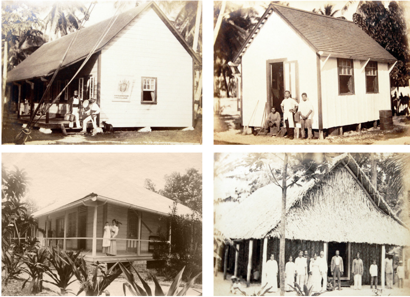
Fig. 4.1: A set of four photographs from Knappe's photographic album. (a), (b), and (c) clearly show prefabricated houses, of which (a) and (b) represent a standardized model without individual extensions, (d) house with traditional palm leaf roofing (private collection Hermann Mückler)
