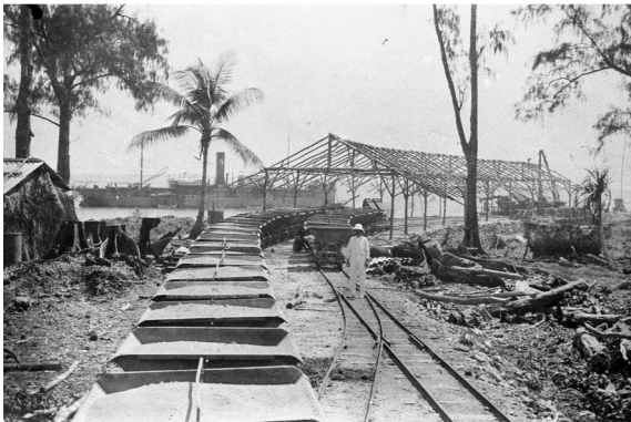
Fig. 5.7: (a): The 'Gute Hoffnungshütte' under construction; (b) Concrete mixing underway in Angaur, the end section of the 'Gute Hoffnungshütte' is visible in the background, c.1912; (c) Preliminary tracks, carts, and loading equipment in Angaur, provided to the Deutsche Südseephosphat Aktiengesellschaft by F. H. Schmidt. A Lloyd steamer waits to be loaded in the background, c.1908 (Deutsches Bundesarchiv, Sammlung Heinrich Hagedorn, Bilder 223–227; 223–046 and 223–046).
