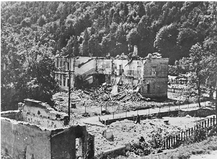
Figure 1: The steelworks in Podbrezová damaged during the war. Source: Betriebsarchiv Stahlwerk Podbrezová.
