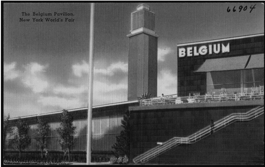
Figure 3.4 Belgian Pavilion, Léon Stynen, Victor Bourgeois and Henry van de Velde, New York, 1939.
