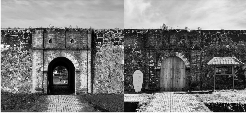
Figure 8.3 Southern gate, also known as the “Waterpoort” with original decorative masonry of red and yellow ijselsteentjes. On the right, the two new information signs are prominently positioned next to the closed doors. Photograph by J. van Donkersgoed, taken on January 31, 2019 and October 10, 2024.
