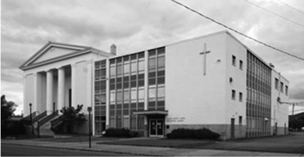
Figure 22.5 Addition to Fourth Baptist Church, Ethel Furman, Richmond, Virginia, 1962.
