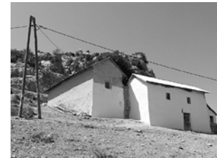
Vernacular architecture in Moulay Bouchta, 2018.
