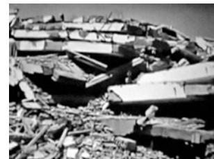
Concrete structures damaged by the earthquake in Agadir, 1960. Stills from Et maintenant Agadir by Louis Roger, 1960.
