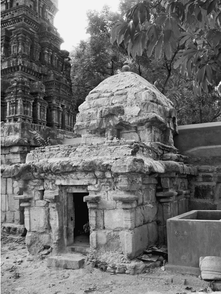
Fig. A.12 Sandstone sub-shrine of Subrahmanya, on the western side of the compound of the AIM (photo by V. Gillet).
