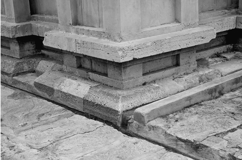
Fig. A.21 South-western corner of the main shrine of the PIM: inscription #41, on the southern façade and #43 on the western façade (photo by V. Gillet).
