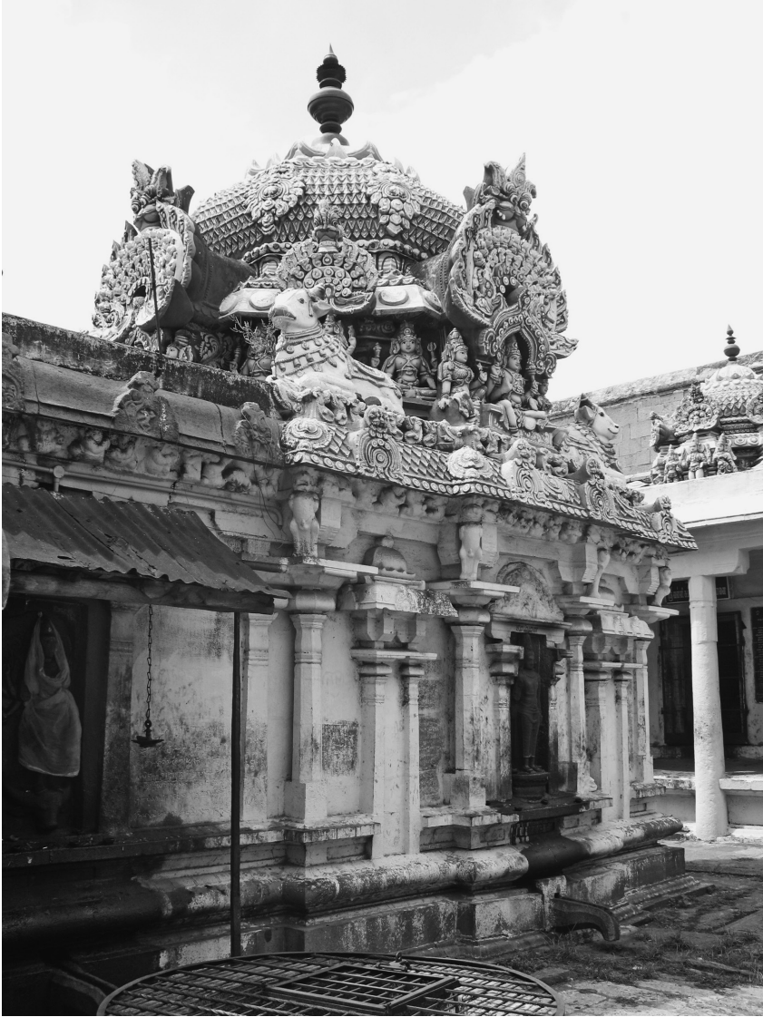
Fig. A.47 Northern façade of the Tiruvālanturai Mahādeva temple (photo by V. Gillet).
