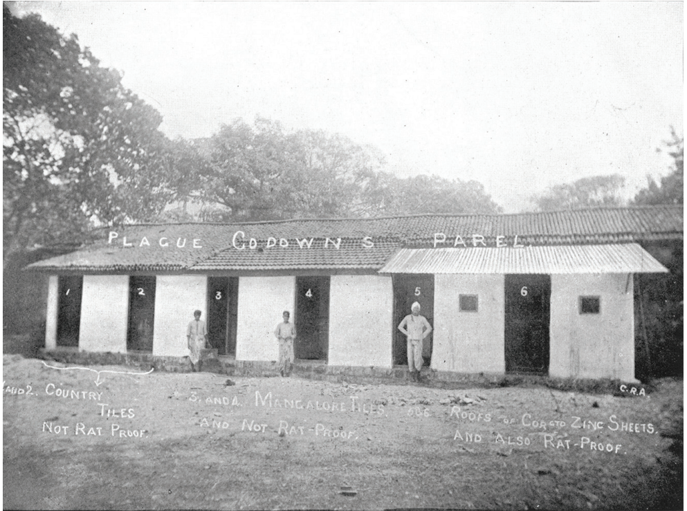
FIGURE 13.1 Photograph of the six “plague go-downs” constructed at the Plague Research Laboratory in Parel, Bombay, designed to mimic different urban structural conditions known to be more or less conducive to plague
